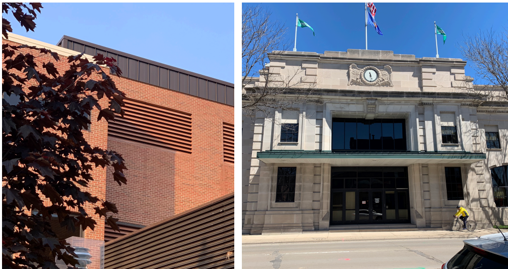
Metal panel on MG&E buildings on S. Blair Street
