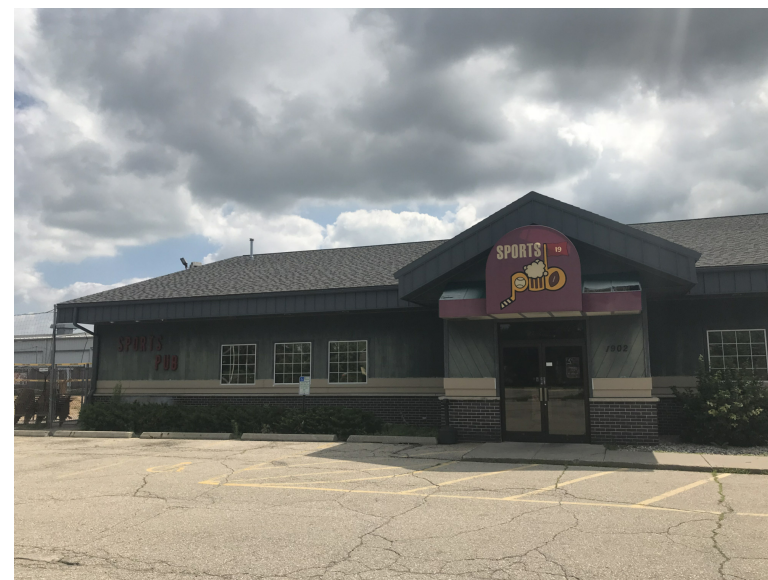
Existing Building West Entry - Looking to NE
