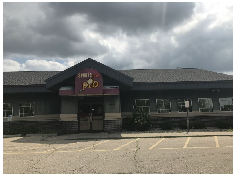
Existing Building West Entry - Looking to E
