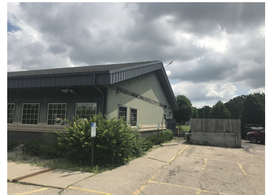
Existing Building South End - Looking to NE
