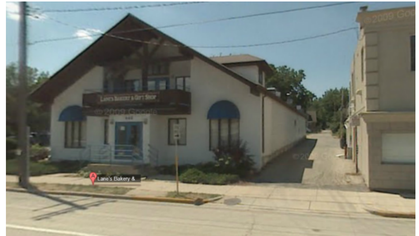
488 S. Park Street (Park Street Elevation - with Alley to right of building)
