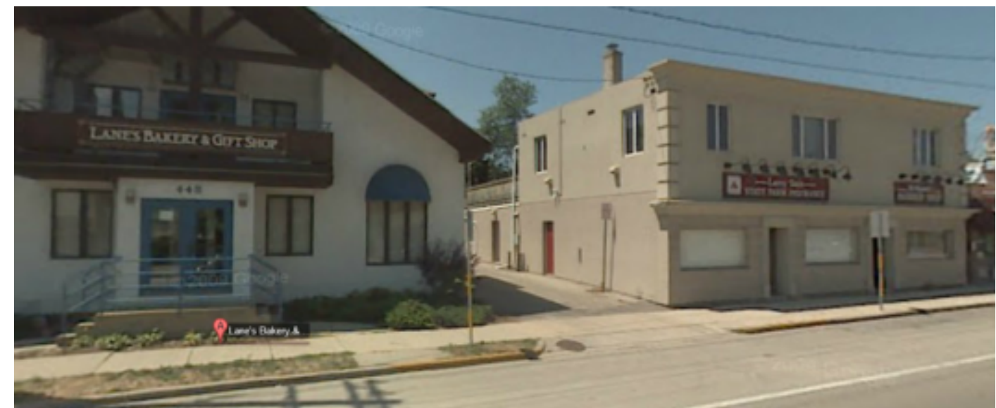
488 S. Park Street & 434 Park Street (Park Street Elevation - with Alley between buildings)
