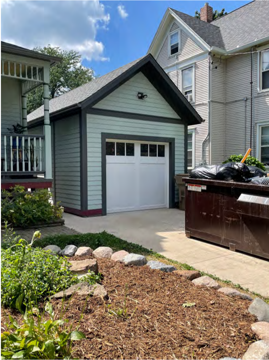
1254 Rutledge, newly built, composite siding, steel garage door
