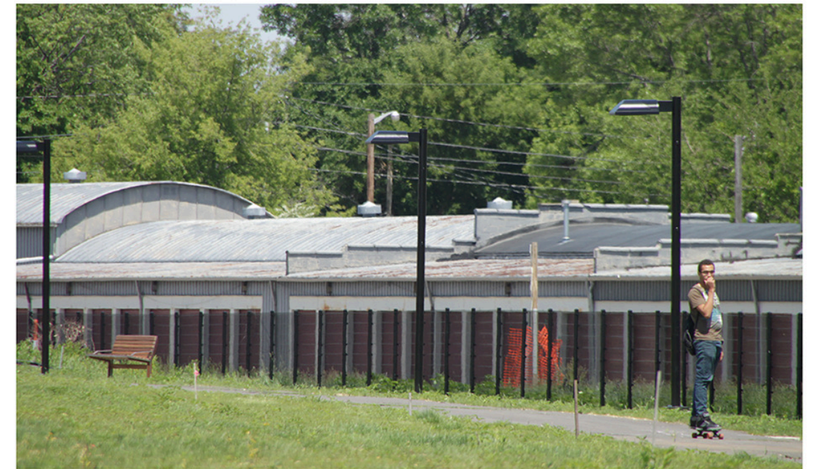
WELDED WIRE FENCE (MATCH CENTRAL PARK)
