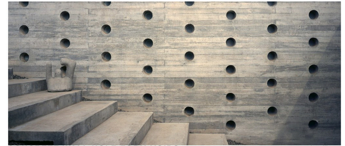
CONCRETE WALL HOLE FORM VOIDS interiii.com
