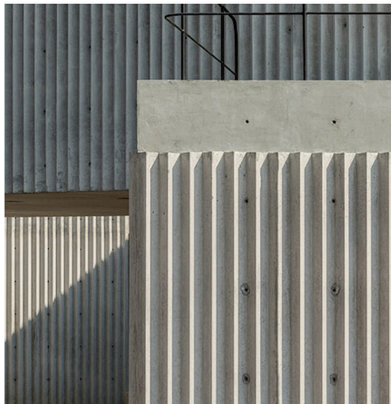
CORRUGATED CONCRETE FORMS housepstudiope.com
