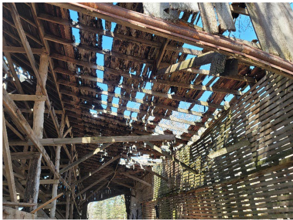
19 – Photo of the roof of the deteriorated roof area of the western barn structure.
