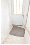
910 Midland Basement Stair.jpg
