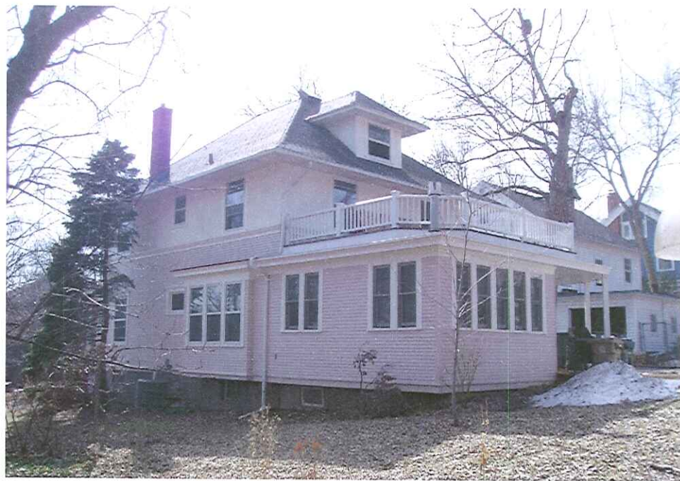
1716 Hoyt - Rear of House
