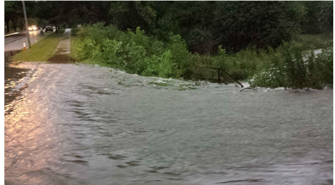
Greenway crossing overtopping at Quarterdeck Dr
