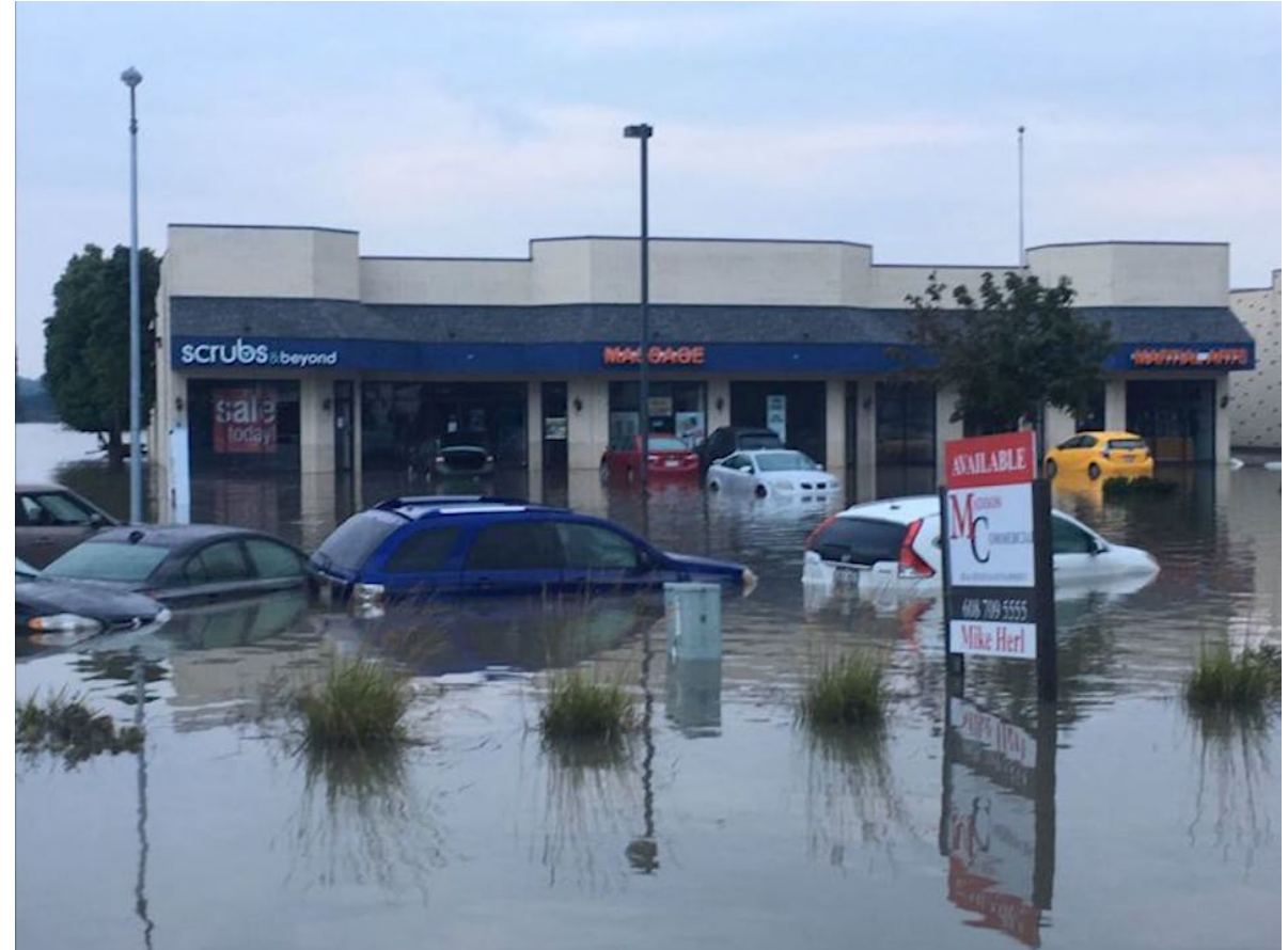
Flooding Near West Towne Pond
