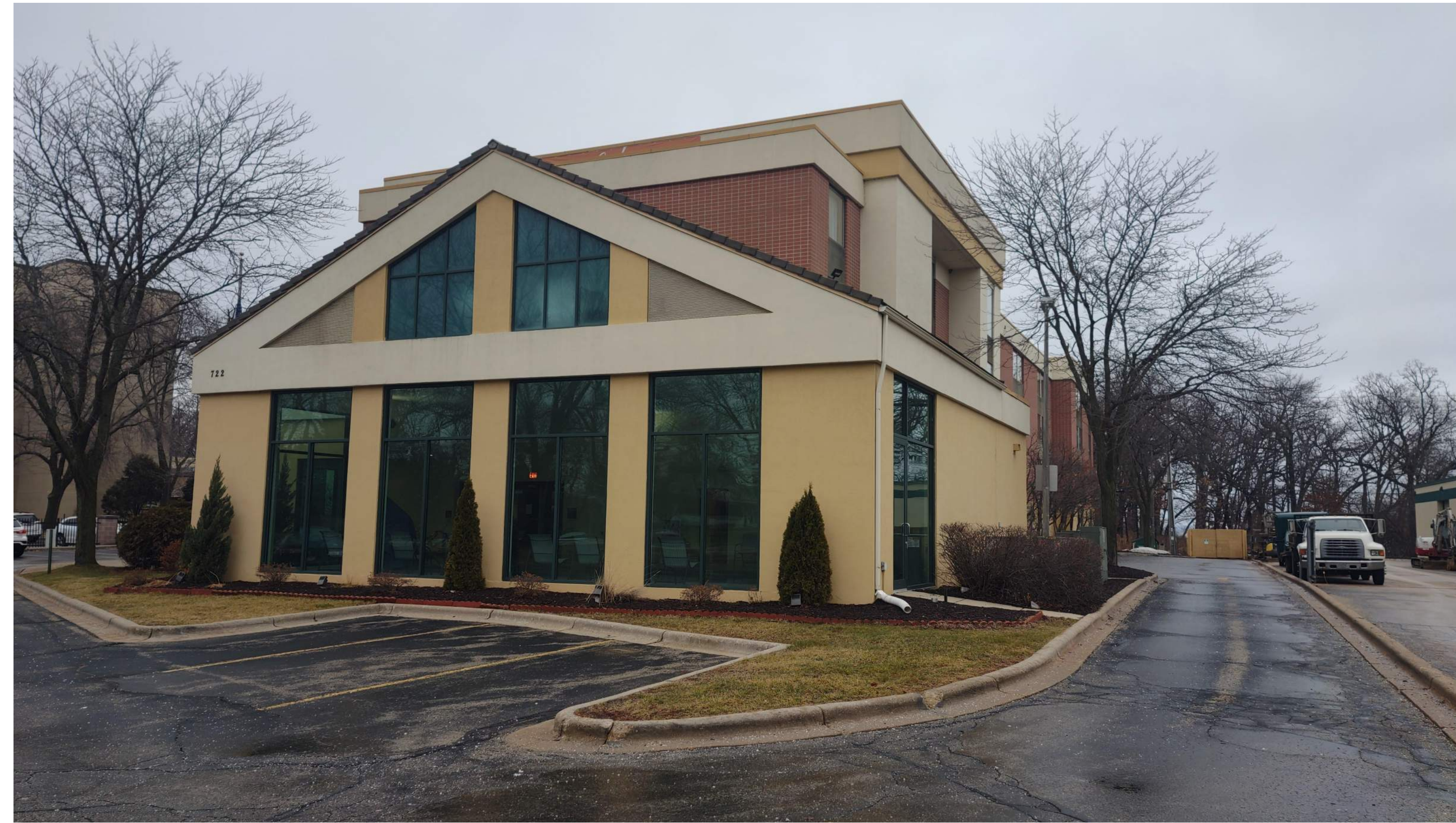
Existing Building Looking North
