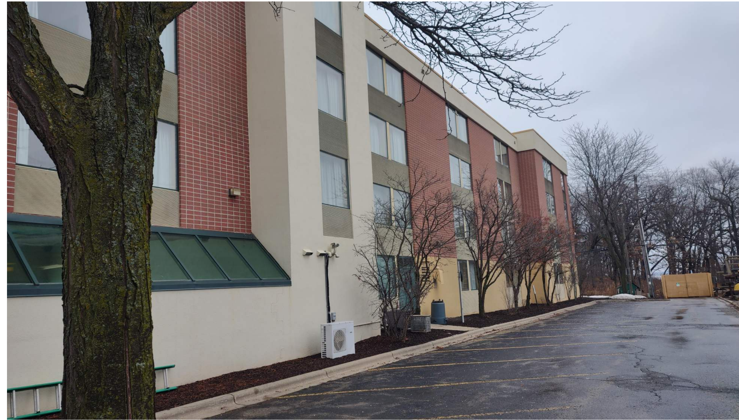
Existing Building Looking North
