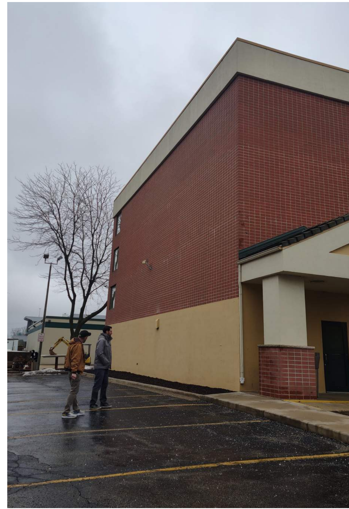
Existing Building Looking West
