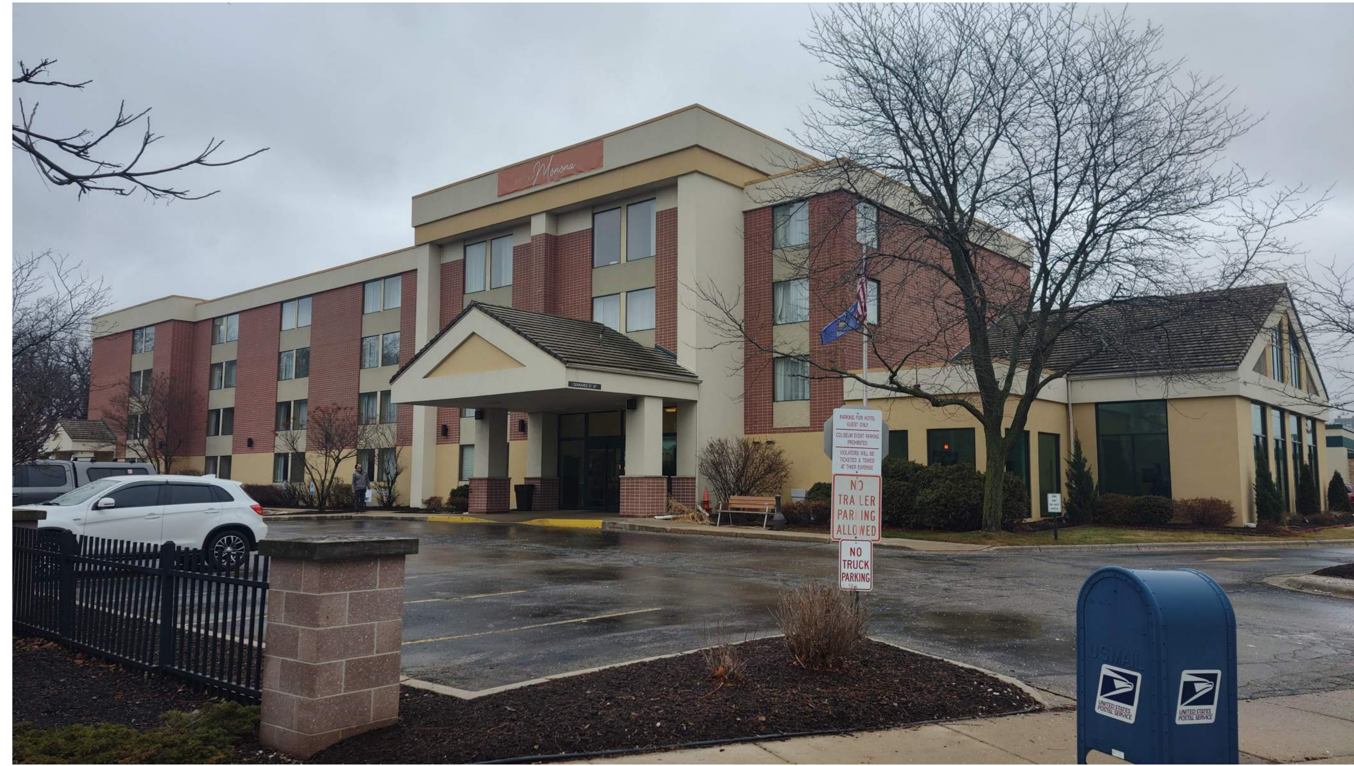
Existing Building Looking East
