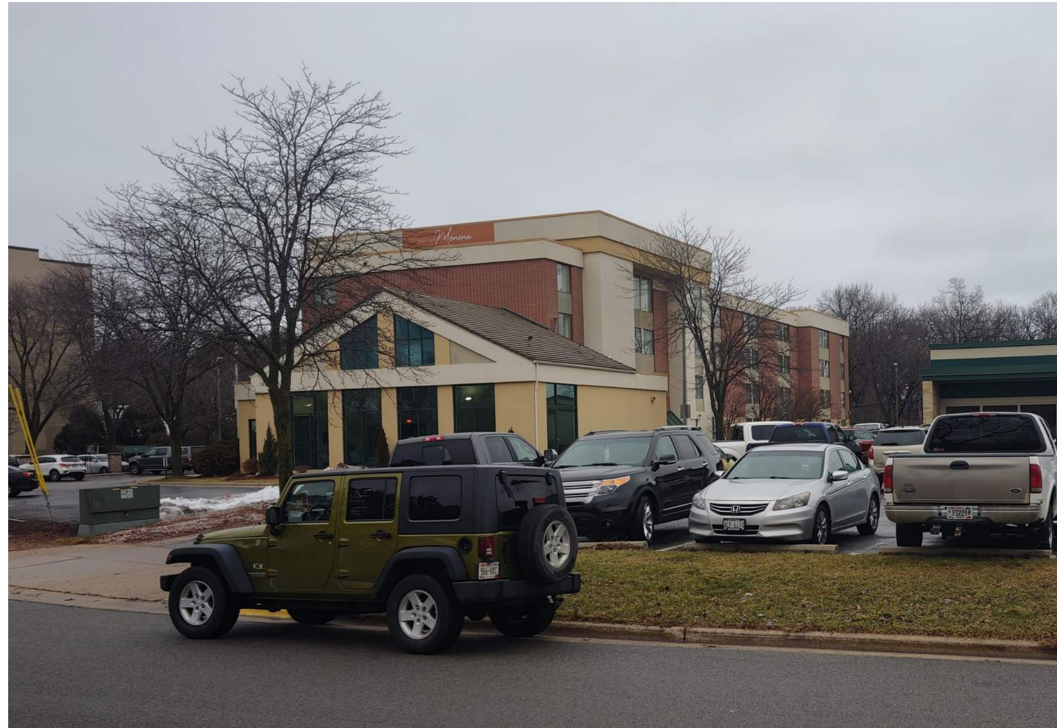
Existing Building Looking North
