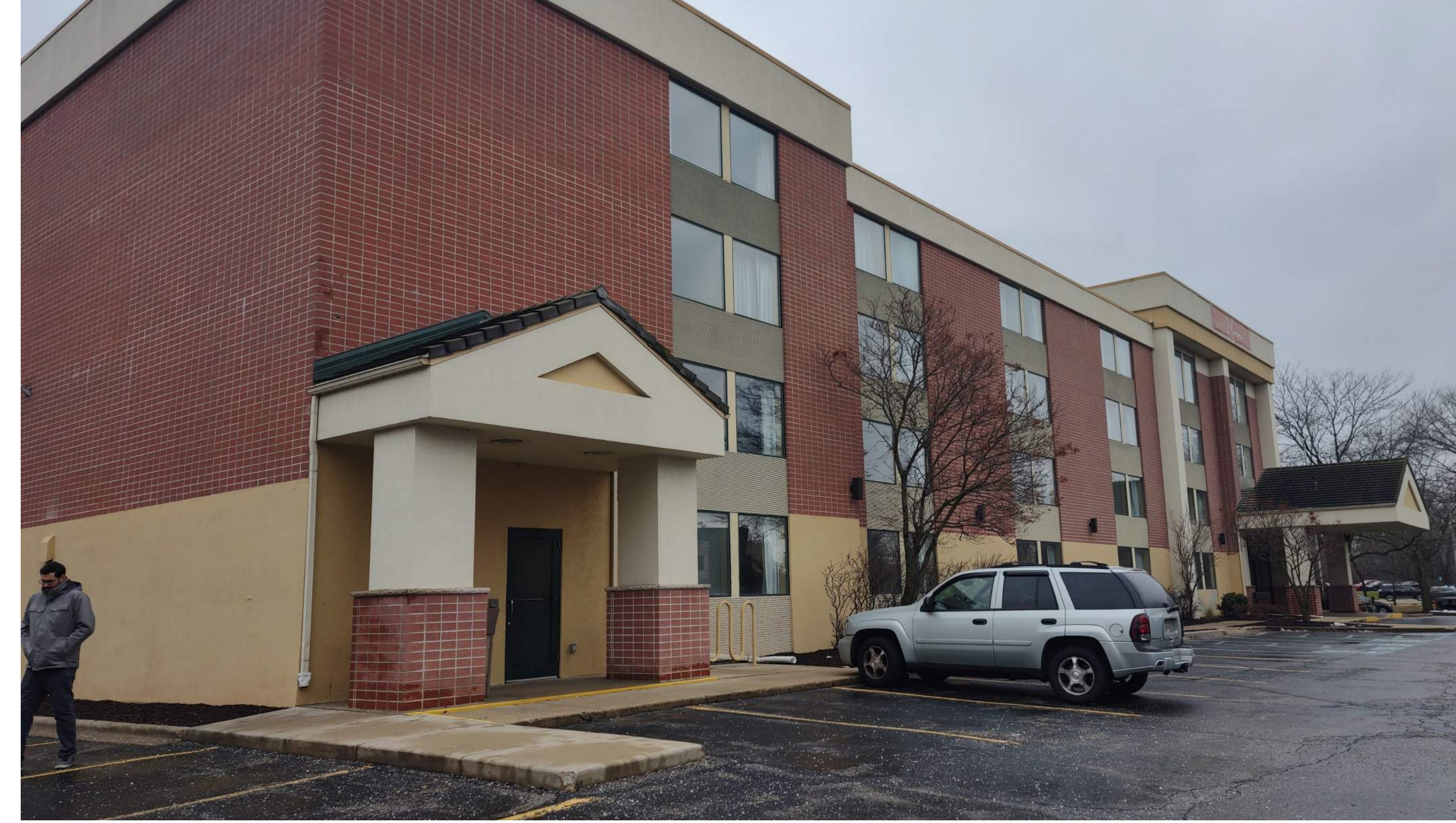
Existing Building Looking South
