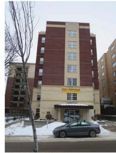
LOOKING TOWARDS THE ROUNDHOUSE AT 614 LANGDON STREET
