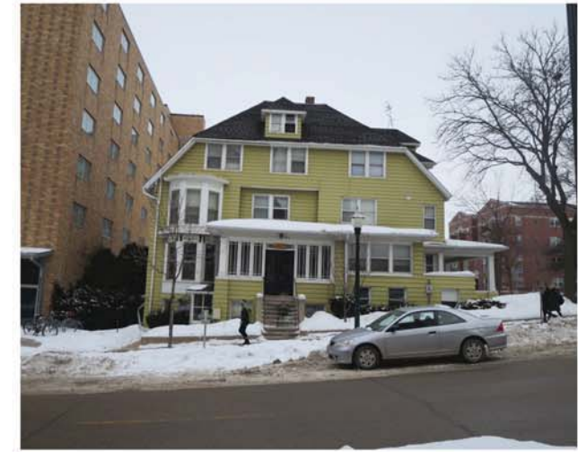
LOOKING TOWARDS THE ROUNDHOUSE AT 602 LANGDON STREET
