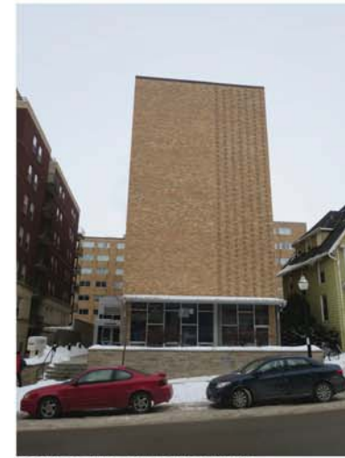
LOOKING TOWARDS THE ROUNDHOUSE AT 610 LANGDON STREET
