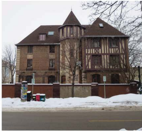
LOOKING TOWARDS THE ROUNDHOUSE AT 636 LANGDON STREET
