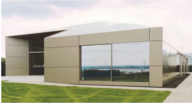
ACM Panel and coping
