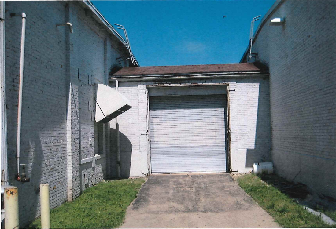
Photo #7 - Site photo looking northwest
