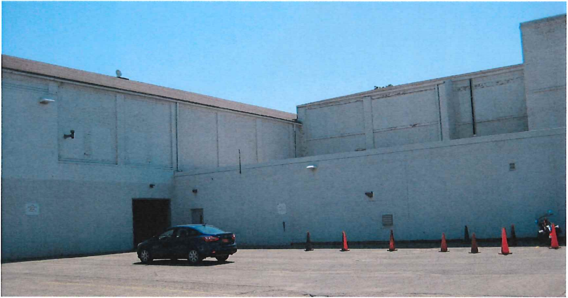
Photo #15 - Site photo looking east
