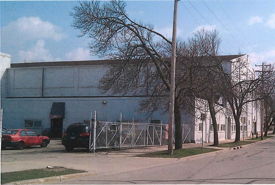
Photo #13 - Site photo looking east
