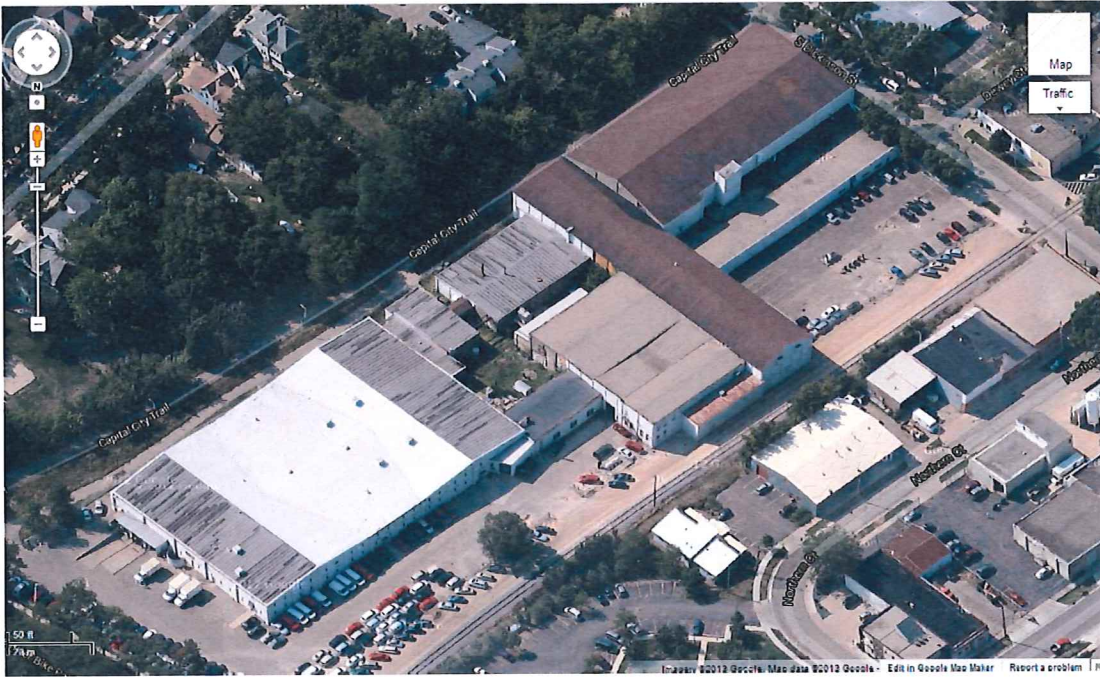
Photo B - Aerial view looking south
