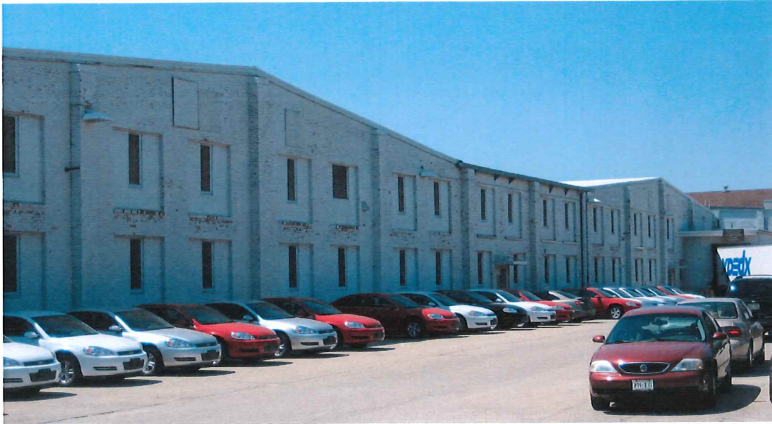
Photo #24 - Site photo looking south
