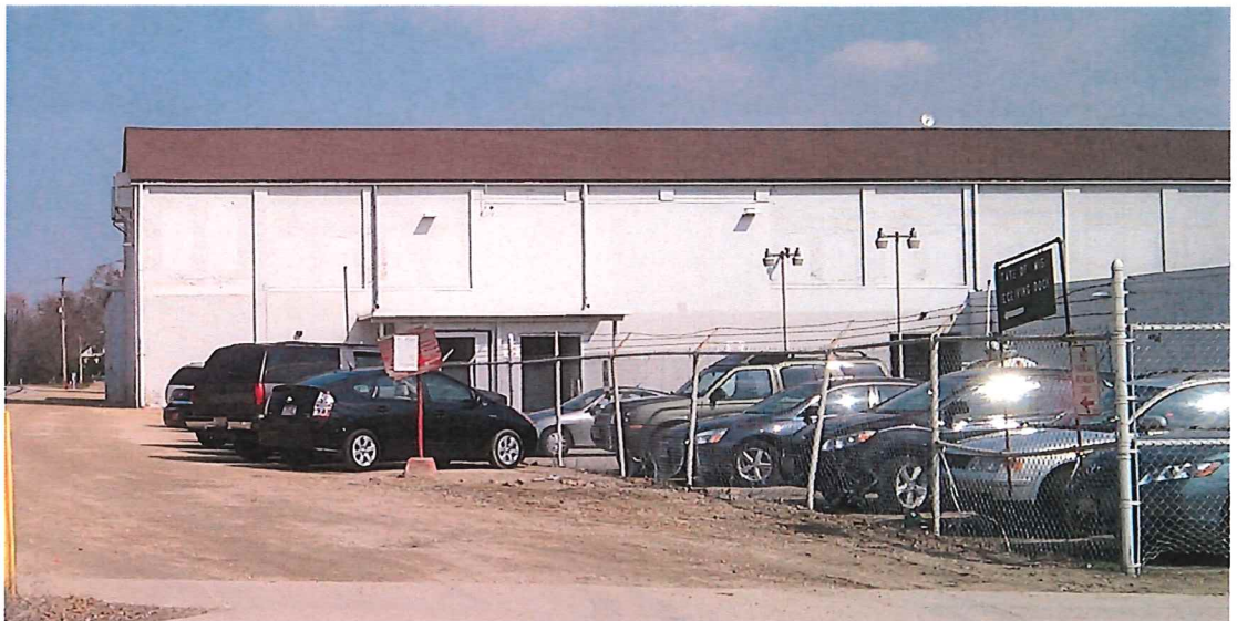
Photo #16 - Site photo looking northeast
