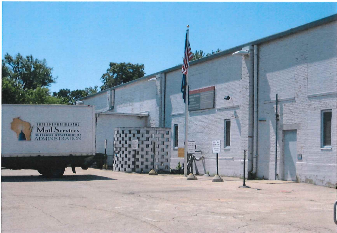
Photo #26 - Site photo looking south
