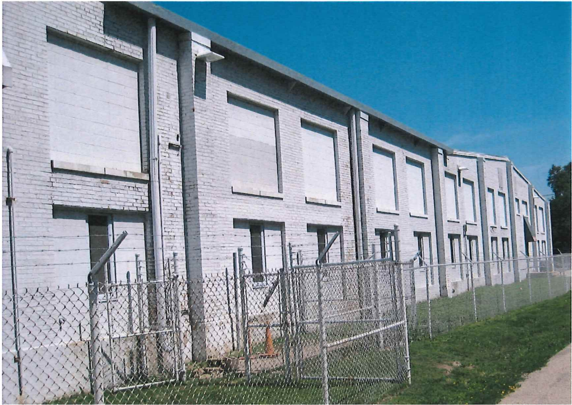
Photo #5 - Site photo looking northeast
