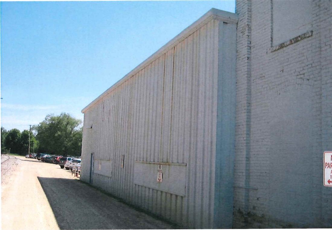
Photo #19 - Site photo looking east
