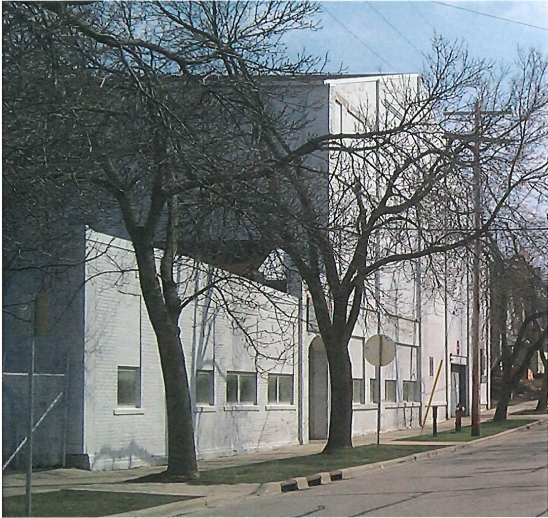
Photo #12 - Site photo looking east
