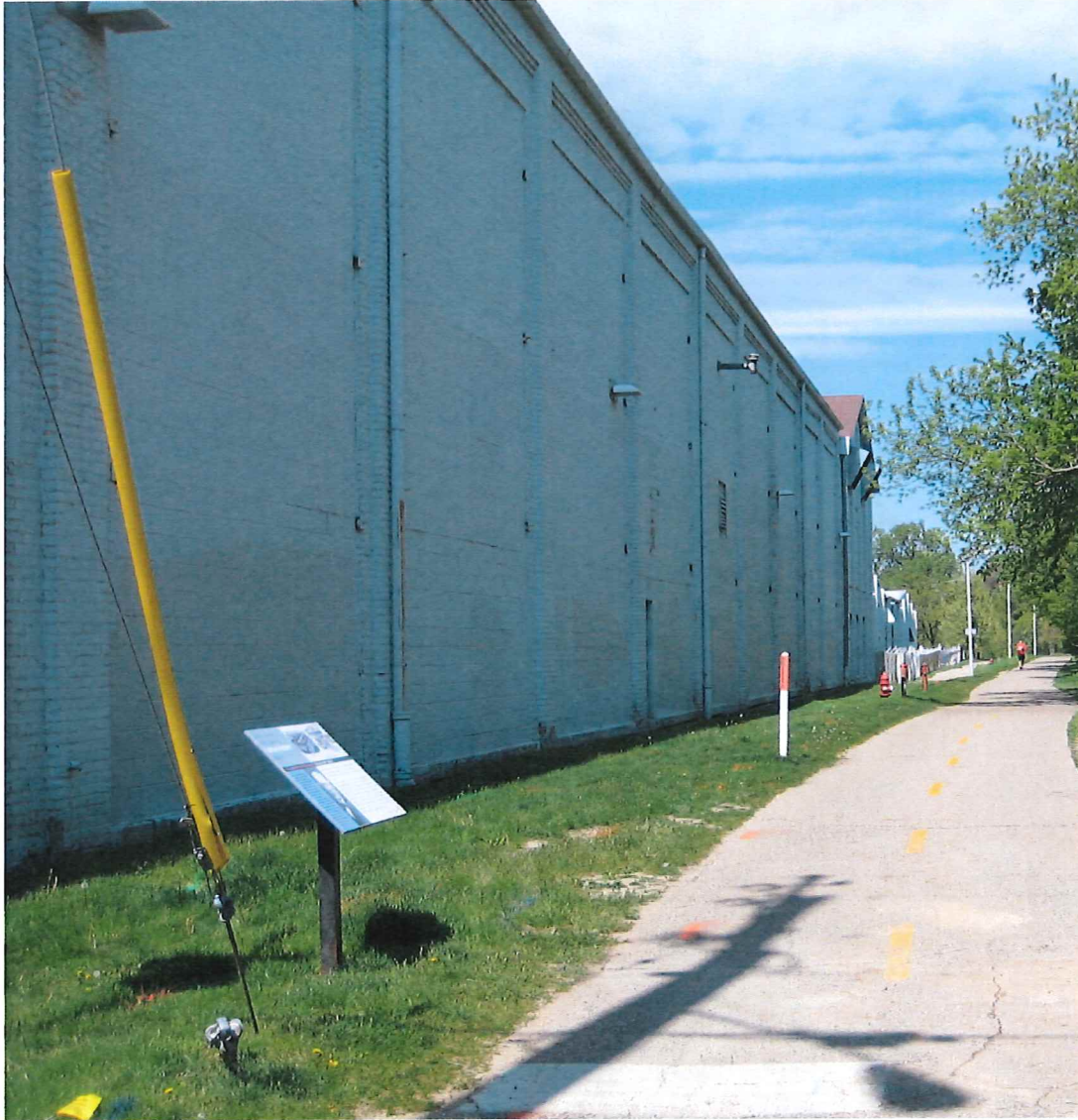
Photo #9 - Site photo looking northeast
