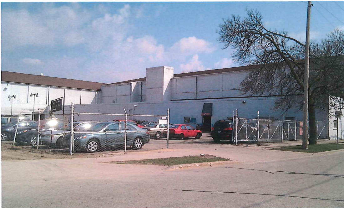
Photo #14 - Site photo looking east
