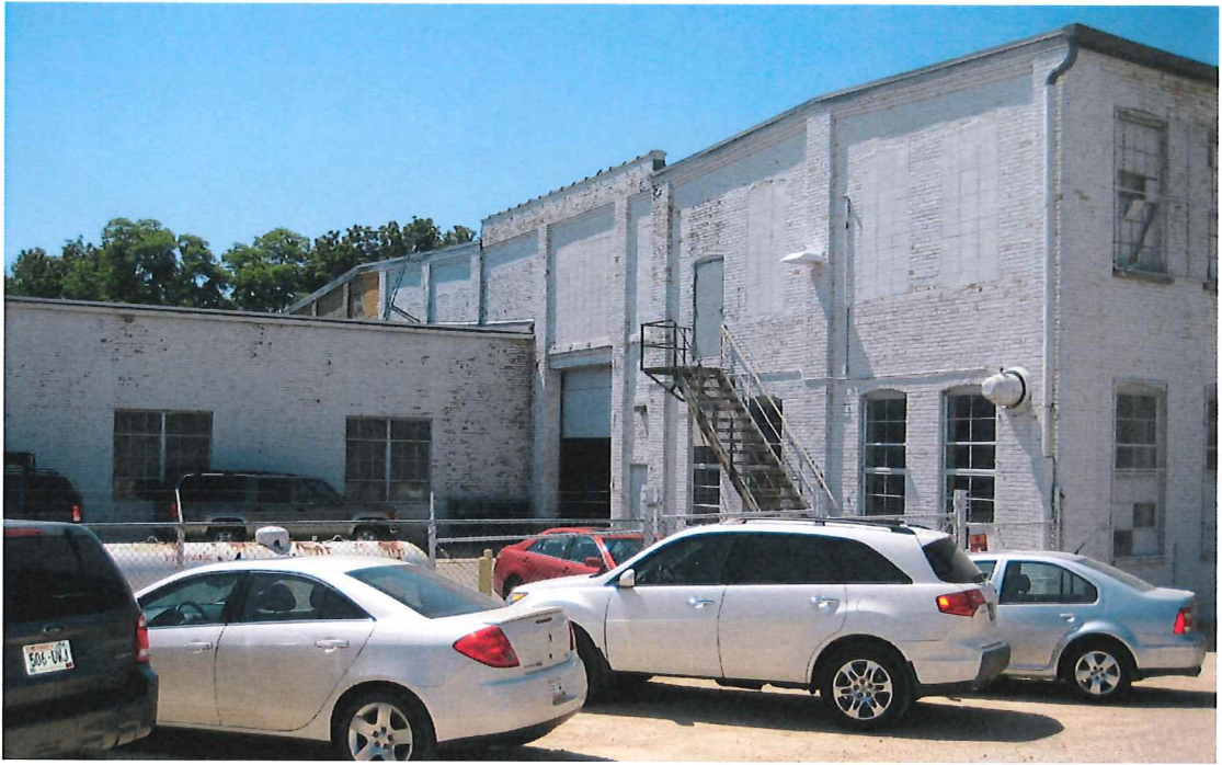
Photo #21 - Site photo looking south
