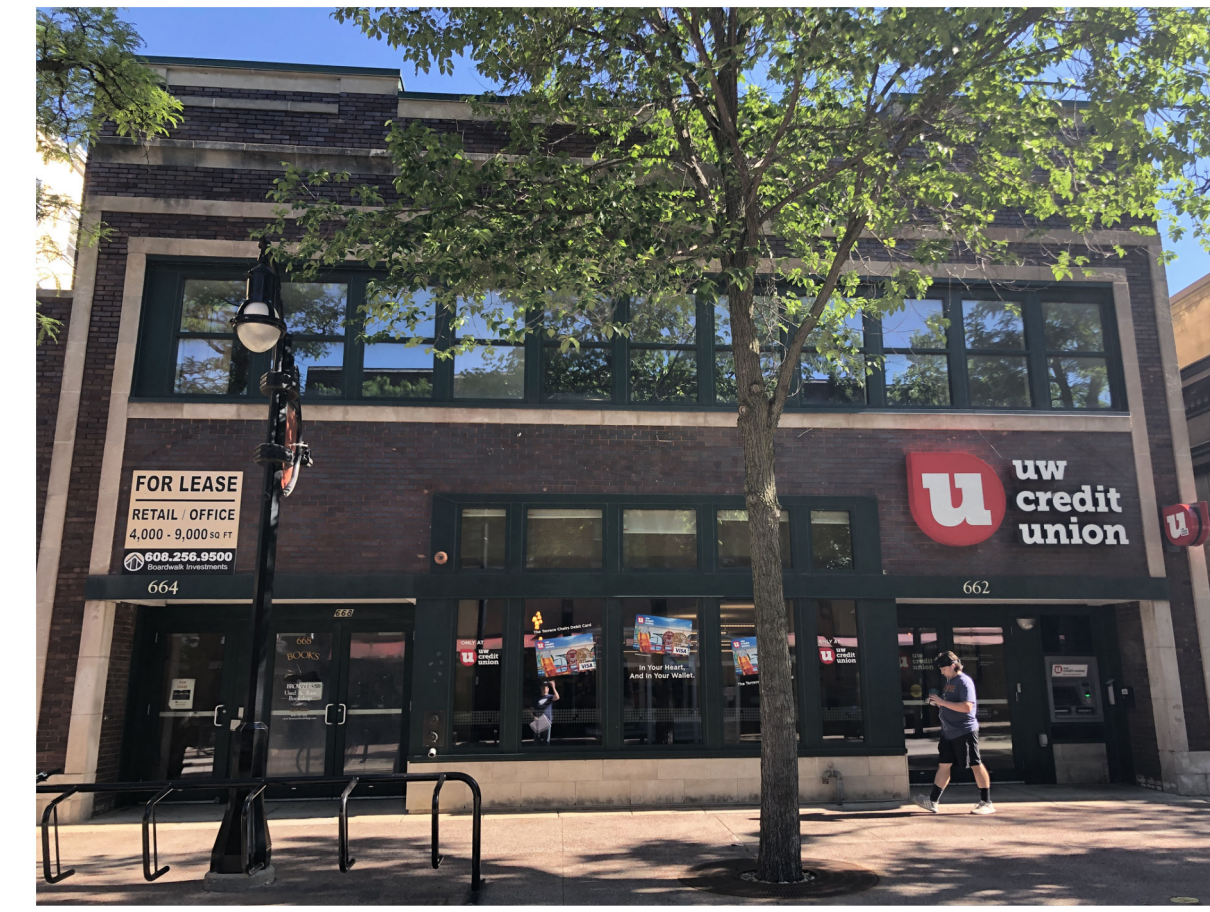
EXISTING PRESENT-DAY PHOTOS (NORTH ELEVATION)
