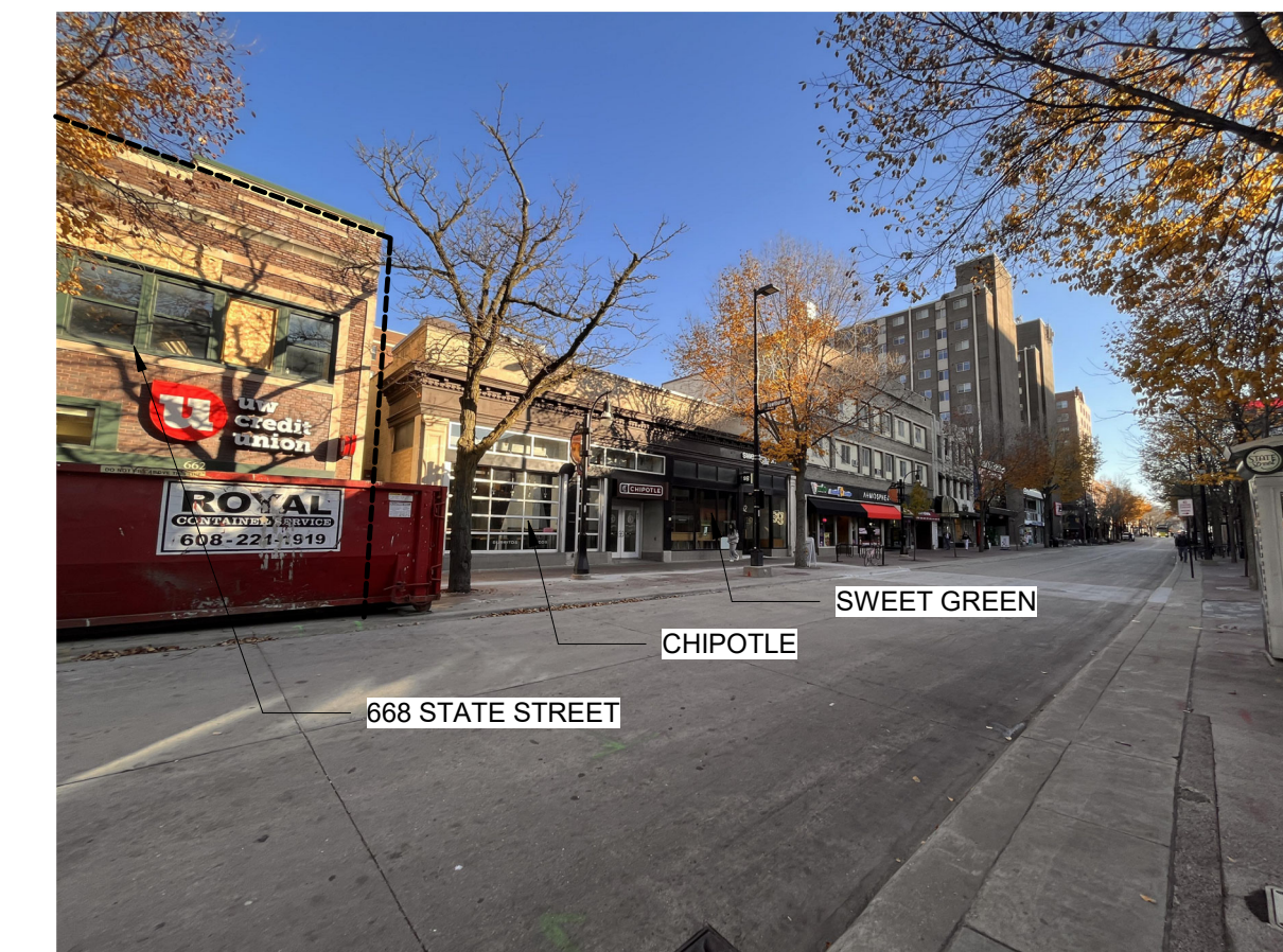
VIEW LOOKING NORTH WEST
