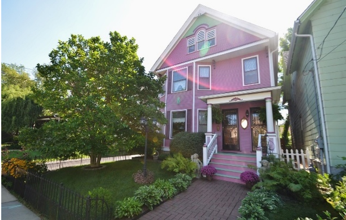
Street front view of home – the primary roof gable is very prominent from this view. This view also shows the close proximity of the neighboring property.
