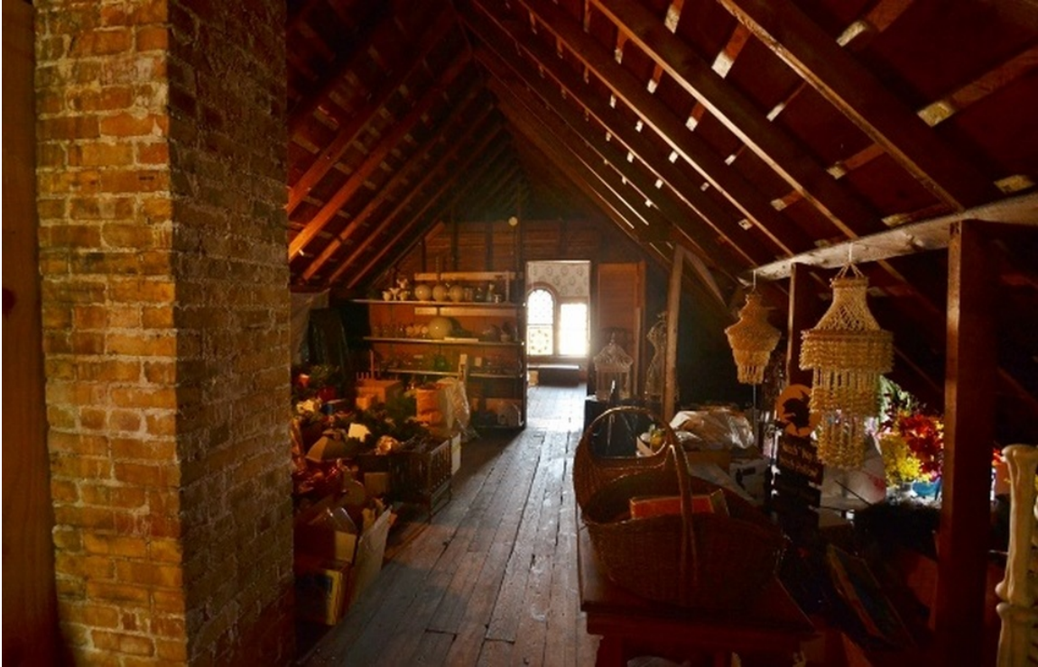
View of the existing unfinished attic space
