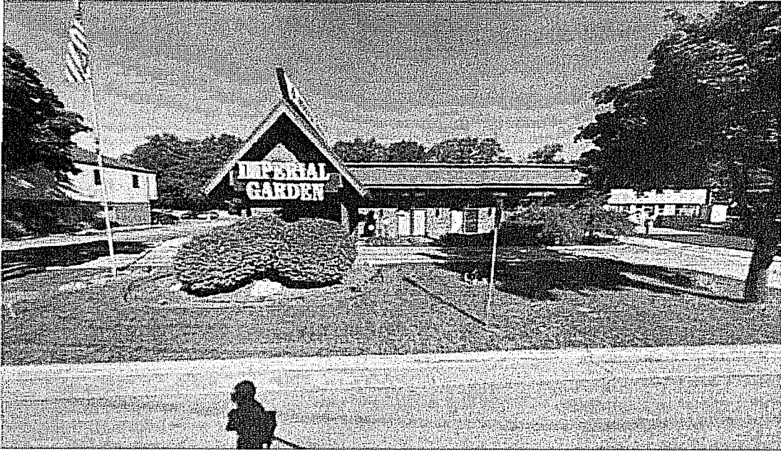
Existing restaurant building on site, as viewed from frontage road.
