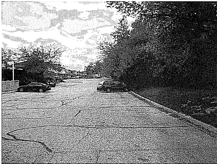
View of rear line, looking southwest
