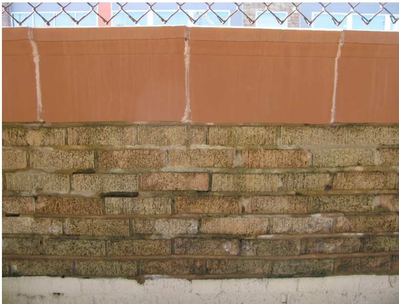
Exterior Wall of 1925 Grandstand
