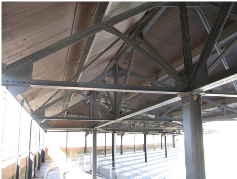
1925 Steel Truss Canopy
