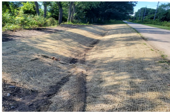
Cannonball Path and Ditch Line Work
