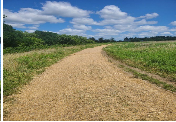
Sycamore Dog Park Path Repair
