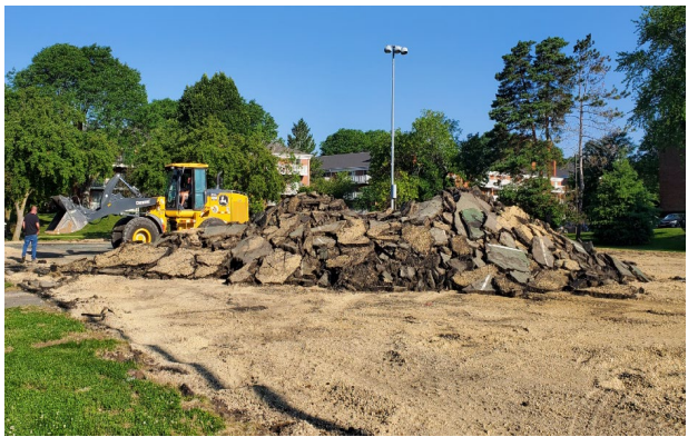
Rennebohm Park – Tennis Court Work
