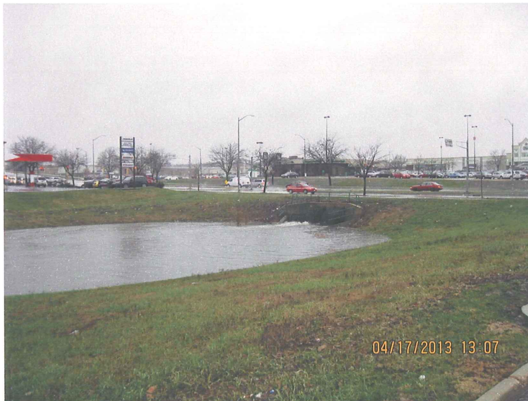
Existing detention pond east of Gammon Road.
