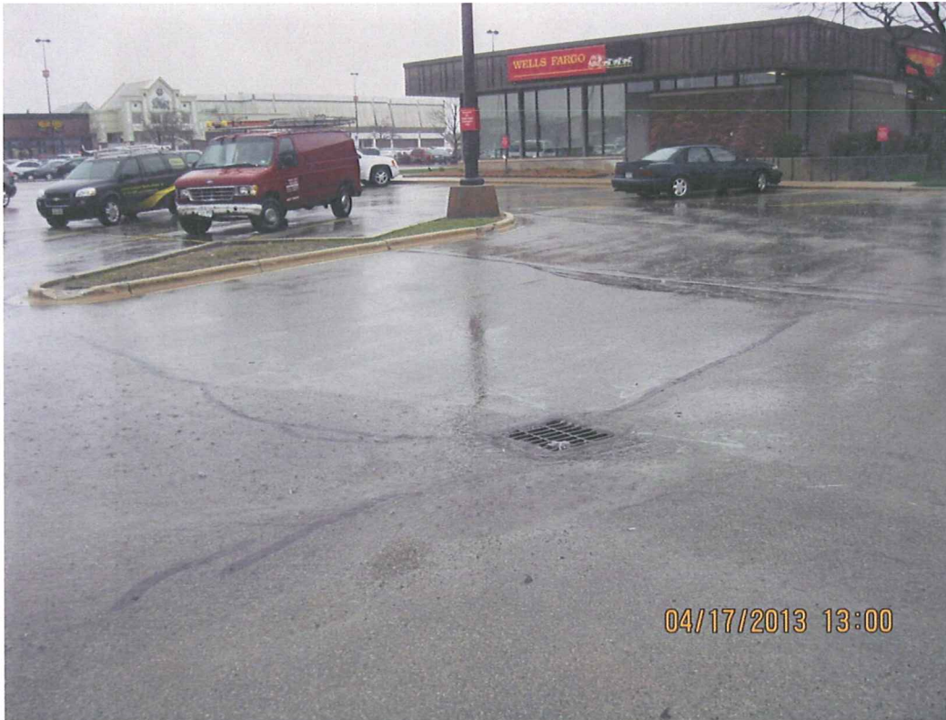
Storm inlet near center of proposed site.
