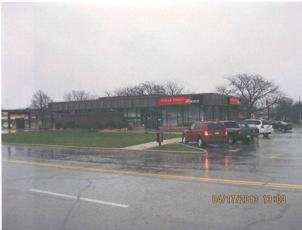
View of west side of existing building.
