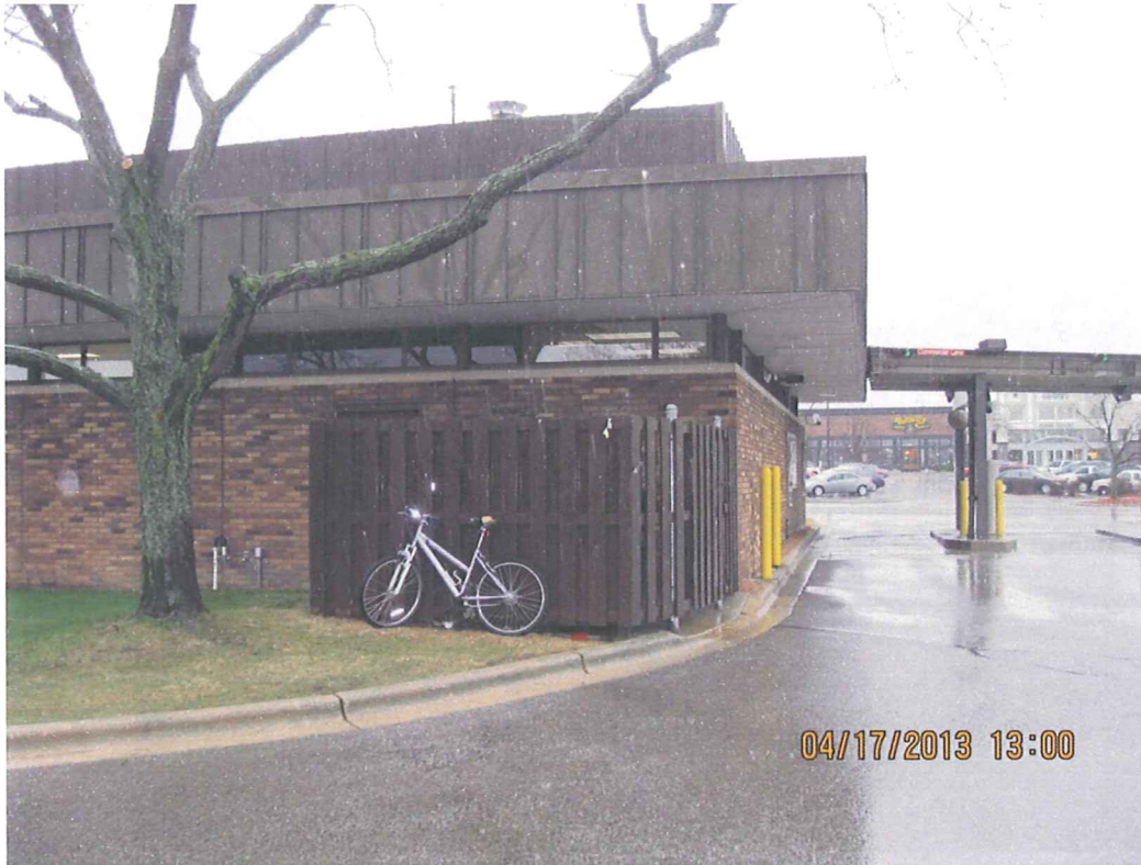
Existing dumpster enclosure and drive-thru.
