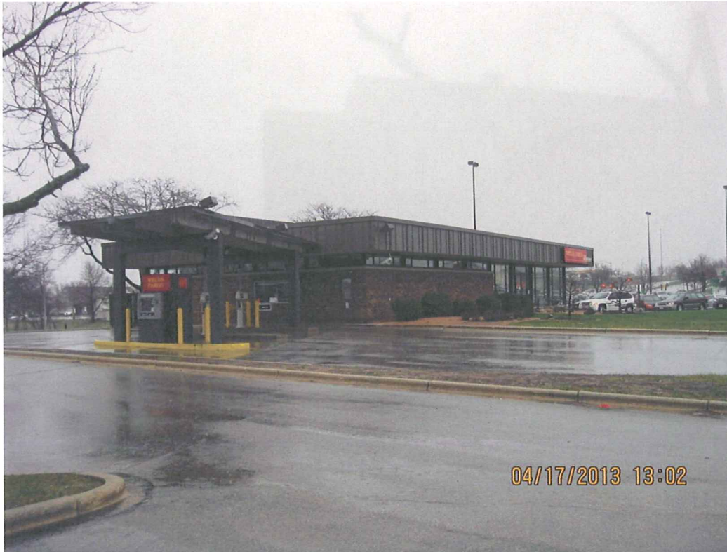
View of northwestern side of existing building and drive-thru.
