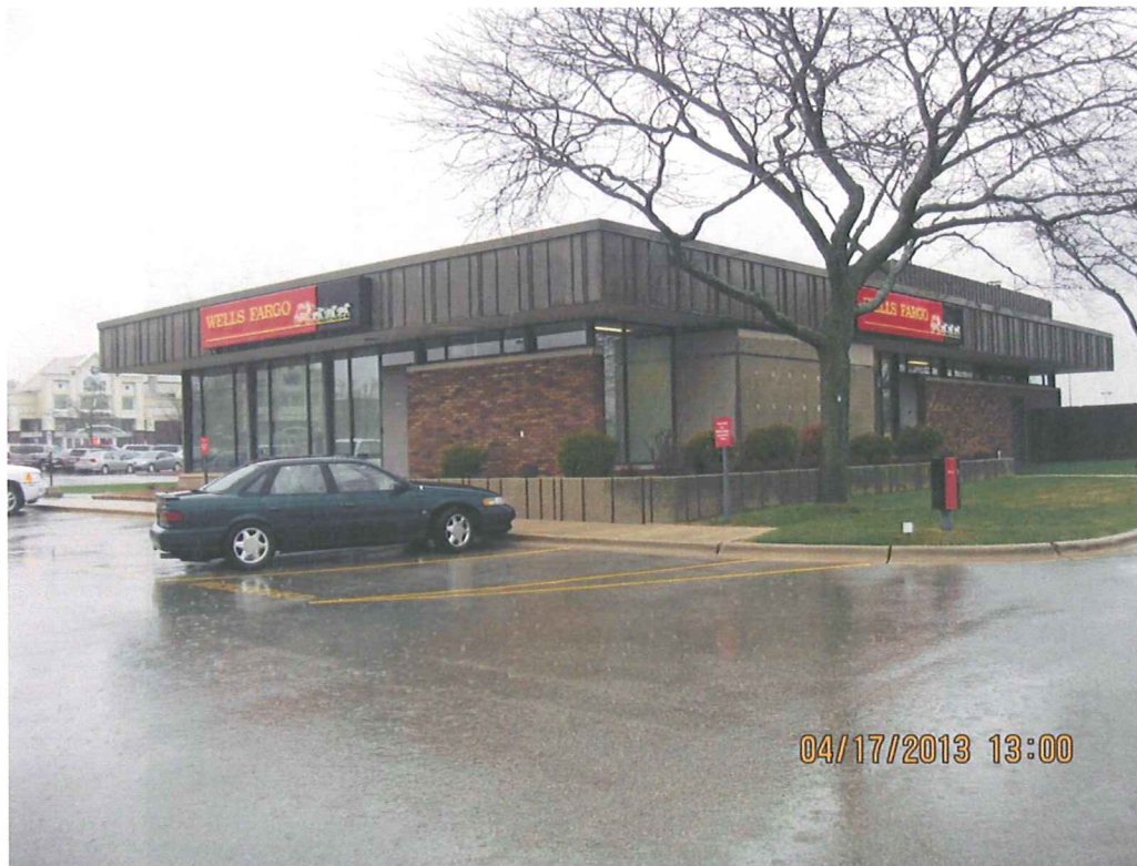
Southeast corner of existing building.
