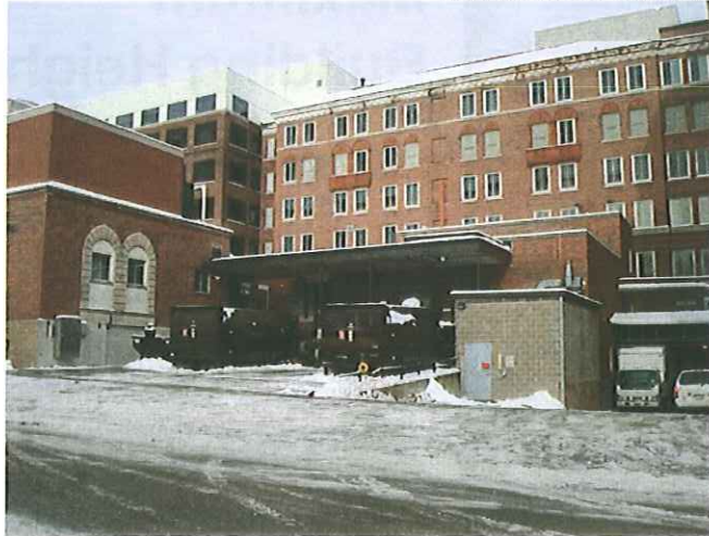
Figure 01: Photo of Existing Loading Area
