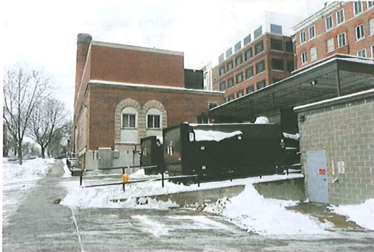
Figure 02: Photo of Existing Loading Area
