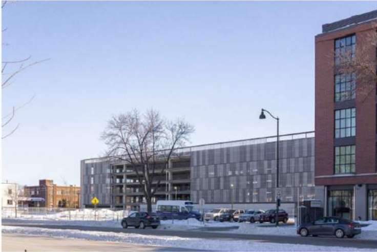
Project site along E. Washington Ave. (Phase 1 Parking Ramp is visible in background)
