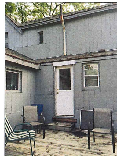
Exterior - Close Up - Back Porch
