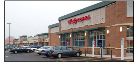
The new Walgreens, improved pedestrian access, new landscaping and additional lighting behind the mall are some of the recent improvements to the Meadowood Shopping Mall .
