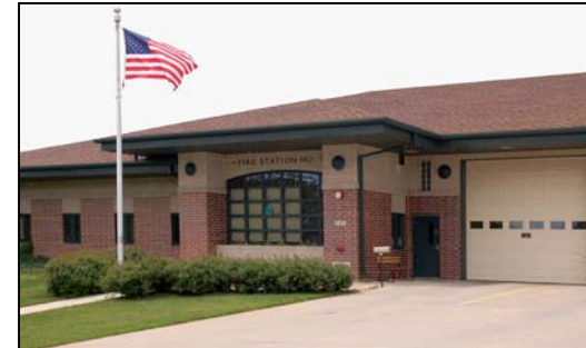
Fire Station 7 provides fire and safety protection for the area. A new ambulance would improve response time for emergencies.
