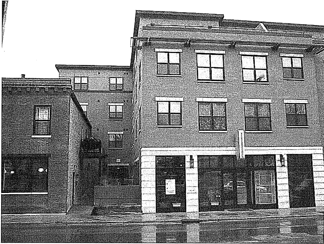
View from Williamson Street. This view shows the entrance to the Market on Williamson Street. It also shows the large overhanging deck in the plaza area. This deck was not in the Plans approved and recorded by the City.
