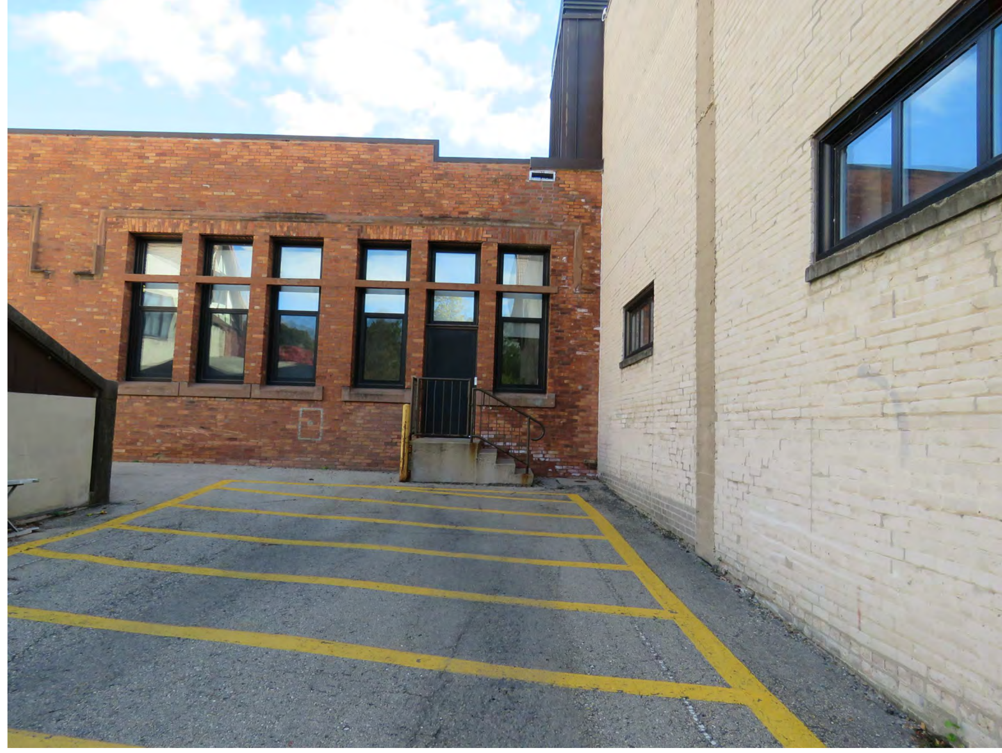
B1 A110 VIEW TOWARDS EXISTING CAFETERIA EXIT & LOCATION OF NEW ADDITION
