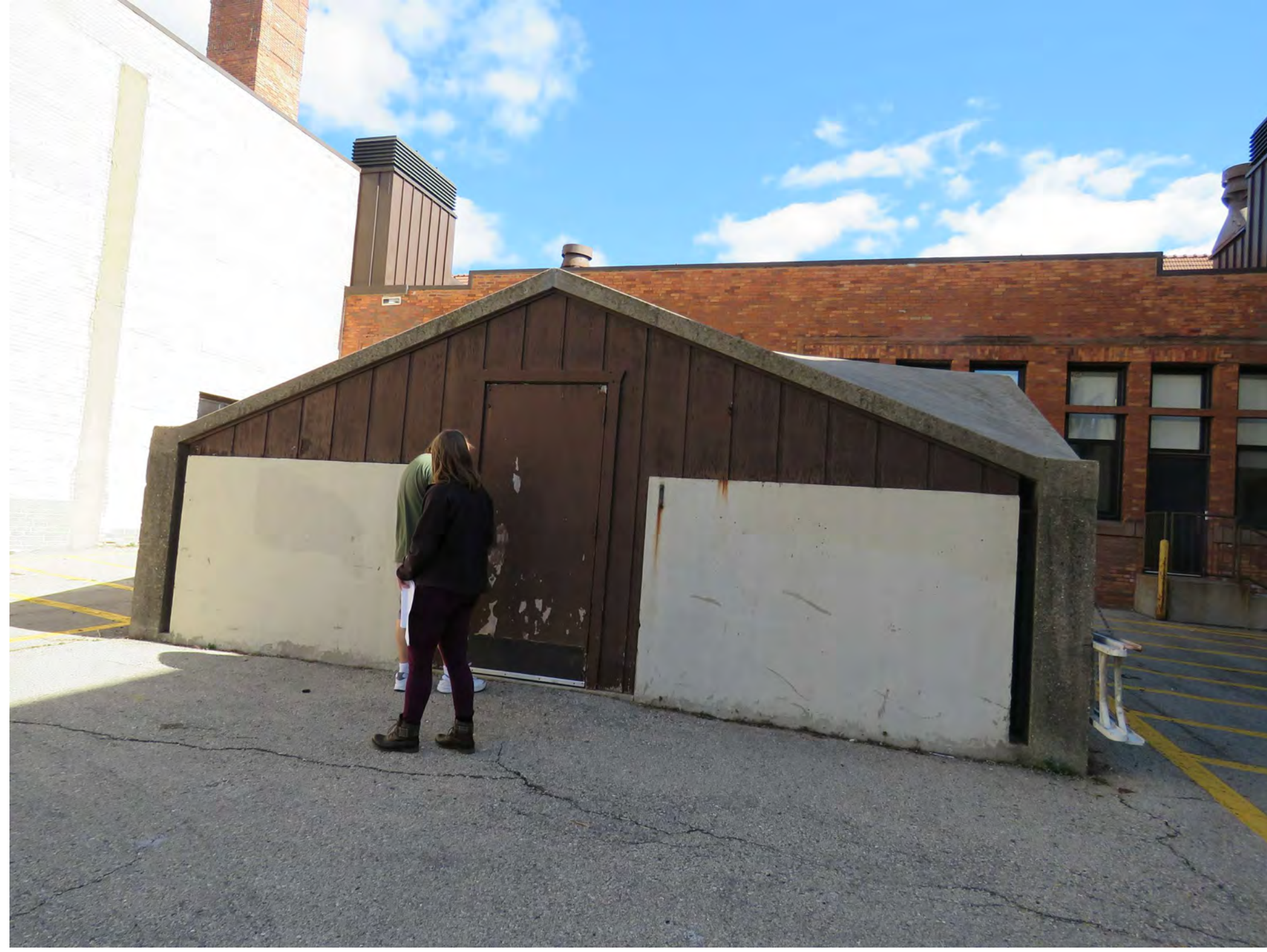
D1 A110 VIEW OF EXISTING MAINTENANCE BUILDING
