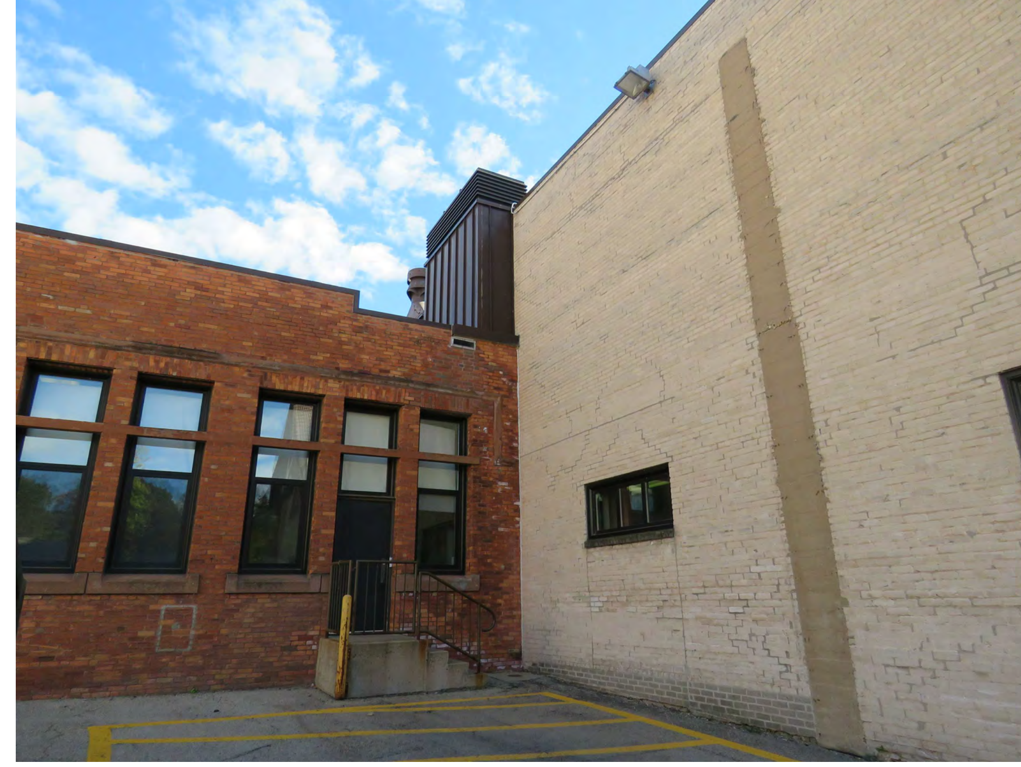
B3 A110 VIEW TOWARDS EXISTING CAFETERIA EXIT & LOCATION OF NEW ADDITION
