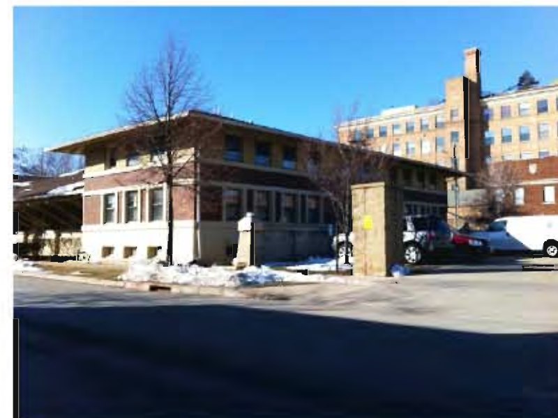
ADJACENT BUILDING ON E MIFFLIN STREET
