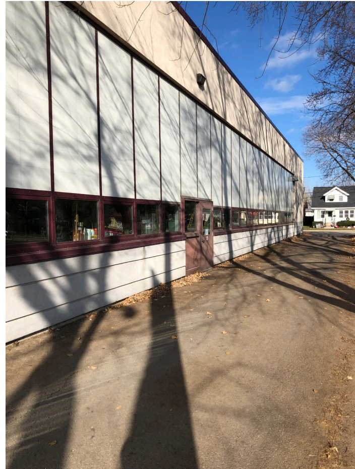
Existing storefront and translucent panel system to be removed
