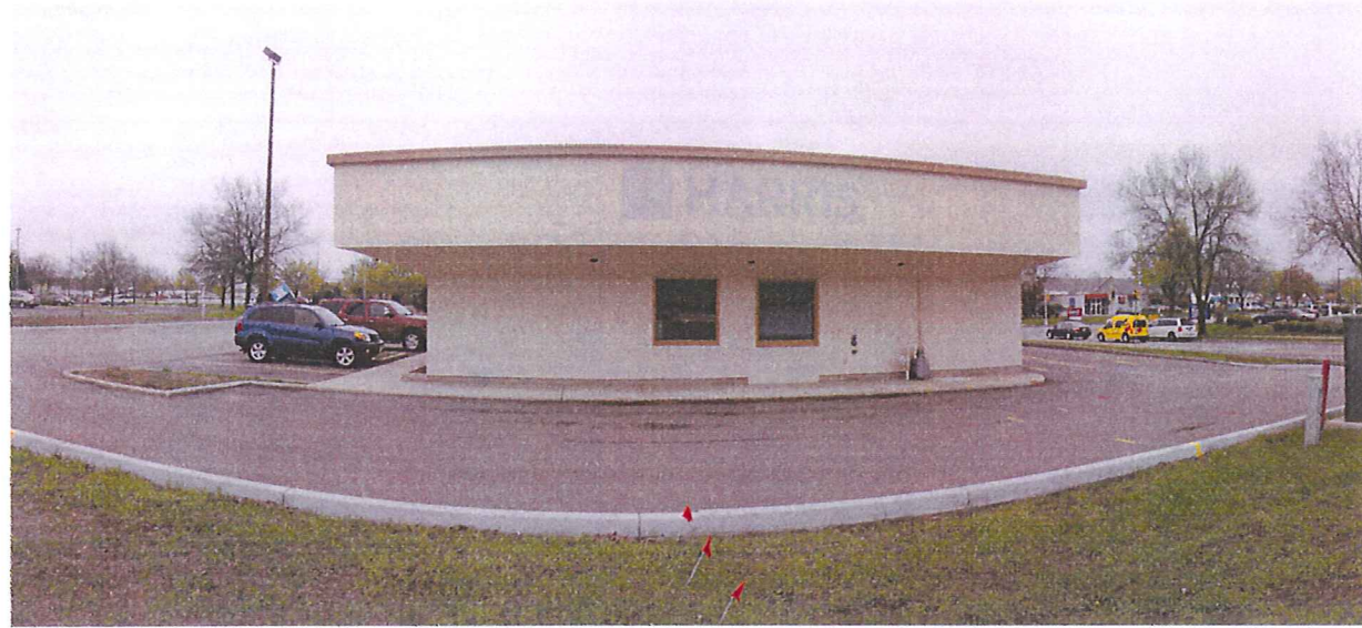
EXISTING BUILDING LOOKING SOUTH
