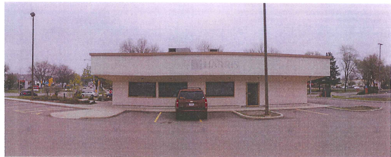
EXISTING BUILDING LOOKING WEST
