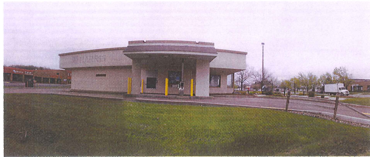
EXISTING BUILDING LOOKING EAST
