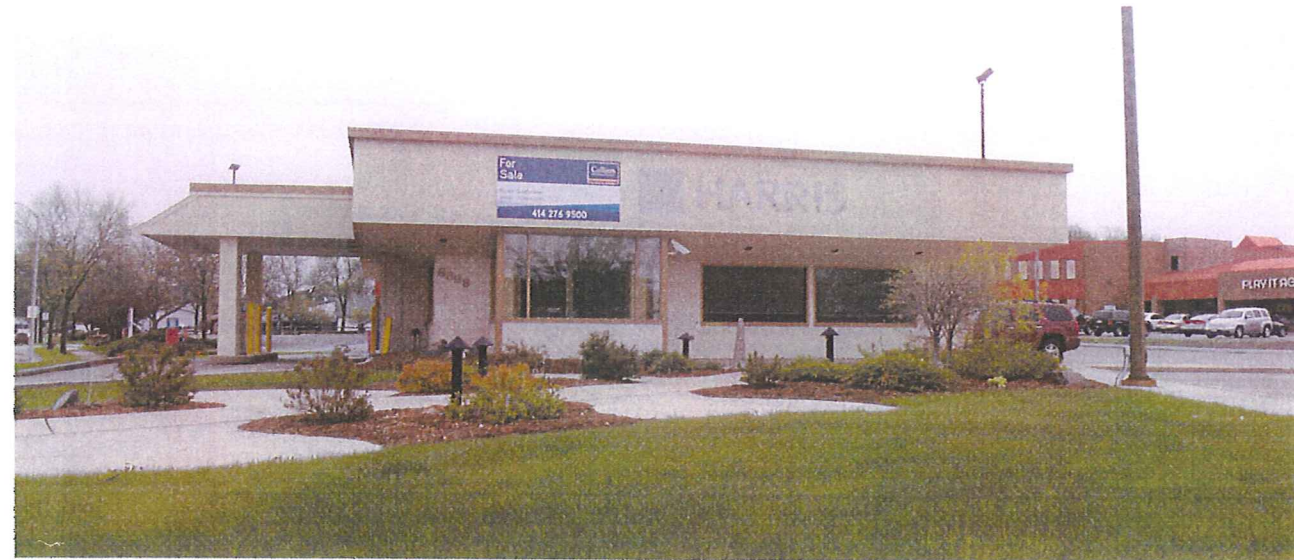
EXISTING BUILDING LOOKING NORTH
