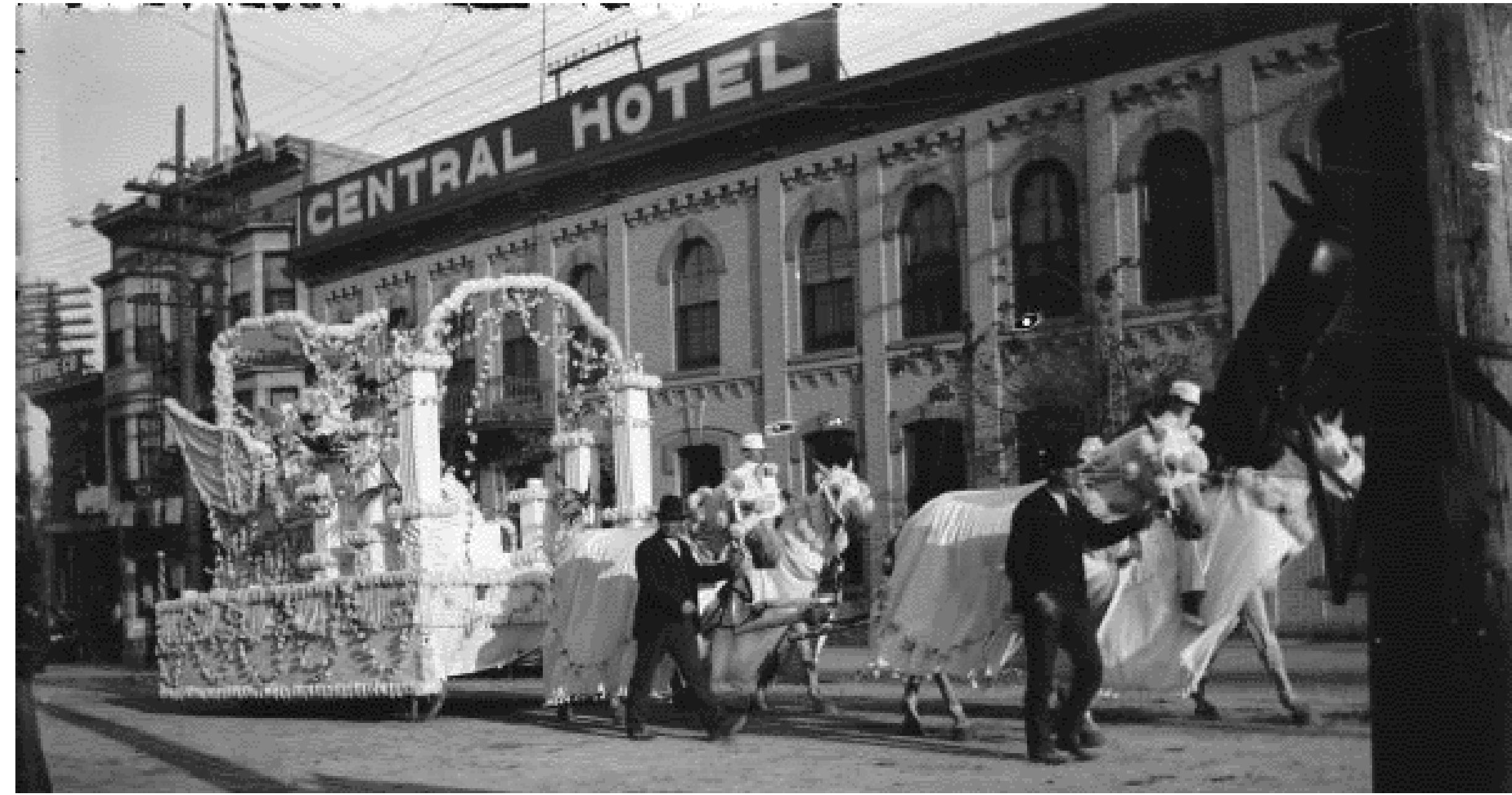
NOTE: REFERENCE PHOTO GRAPH FROM 1905 +/- REMODELED IN 1903 PERIOD OF SIGNIFICANCE = 1825 - 1899
