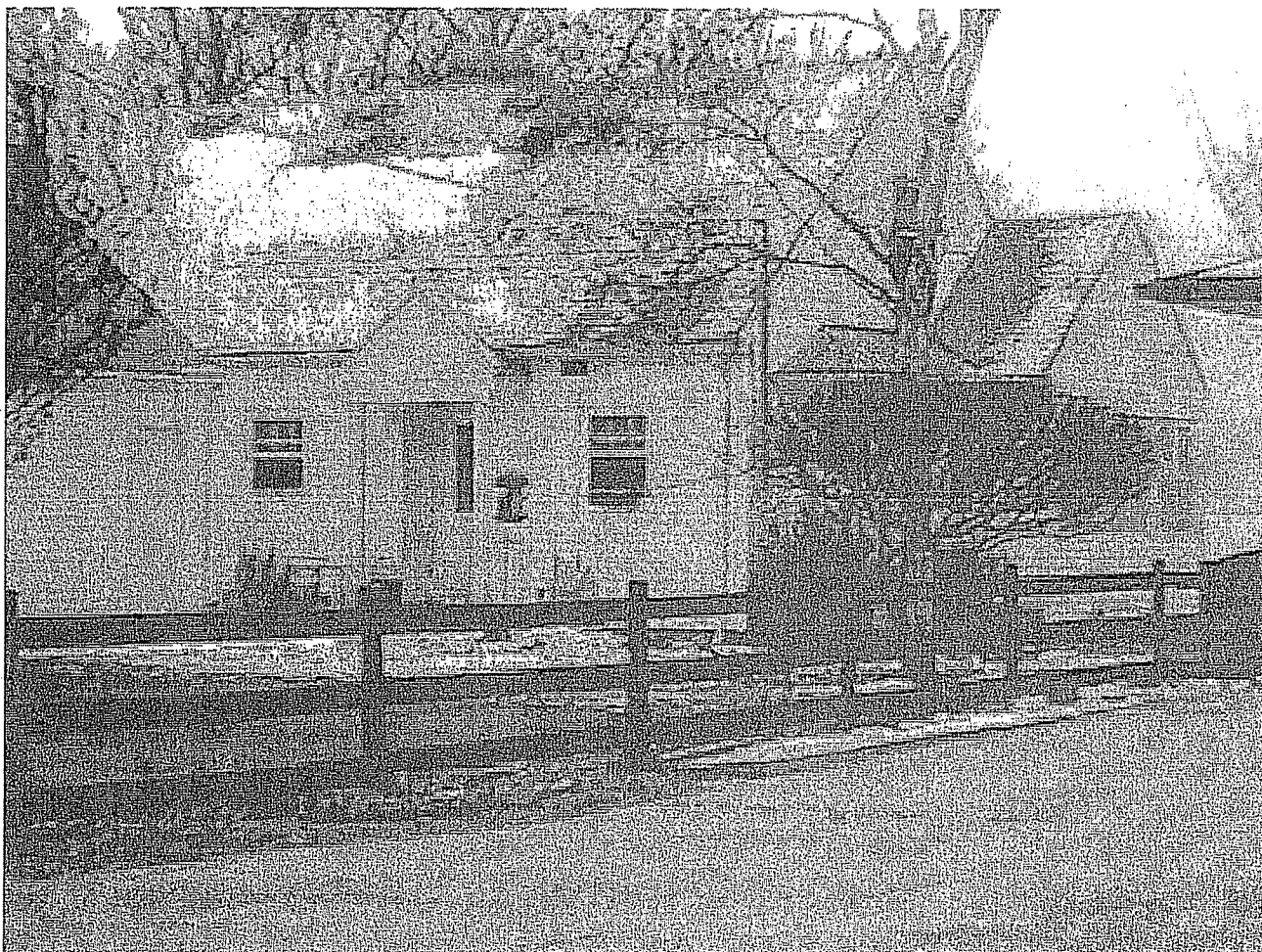
721 Woodward Drive. Proposed for demolition for new house
