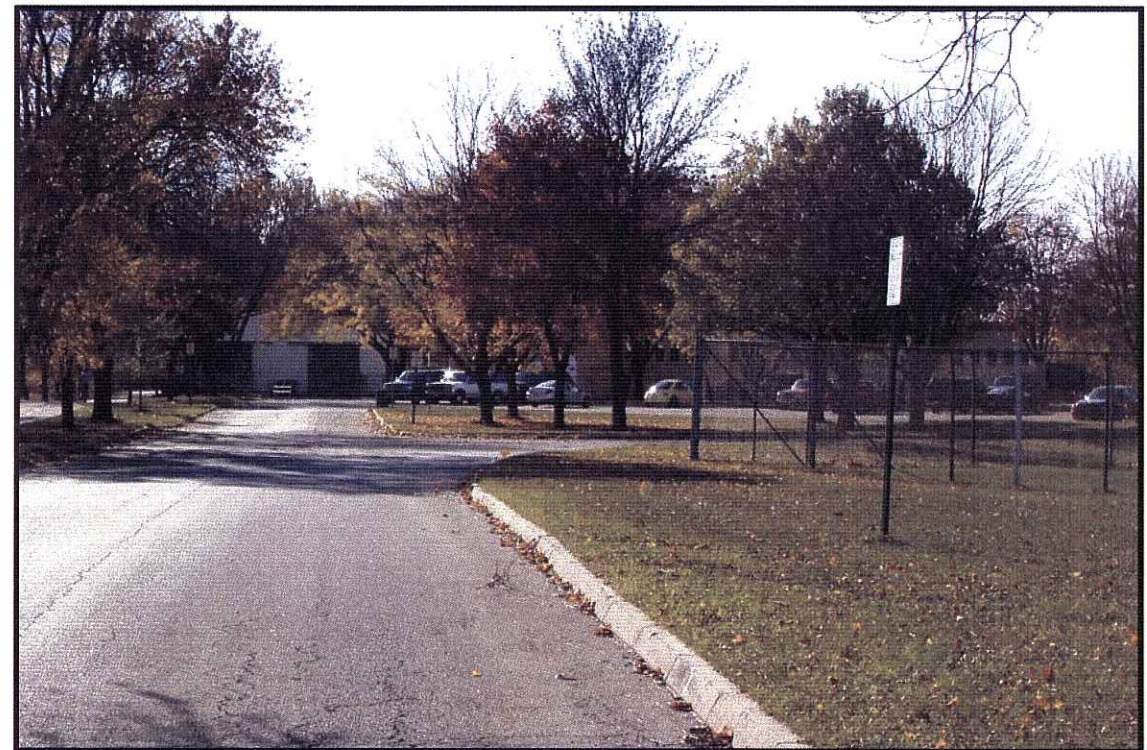
VIEW OF PARKING AREA & MAINTENANCE FACILITY
