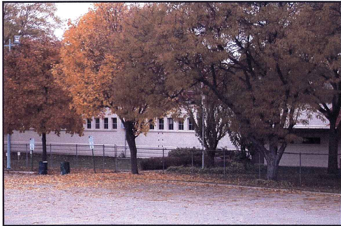
VIEW OF EXISTING MAINTENANCE FACILITY
