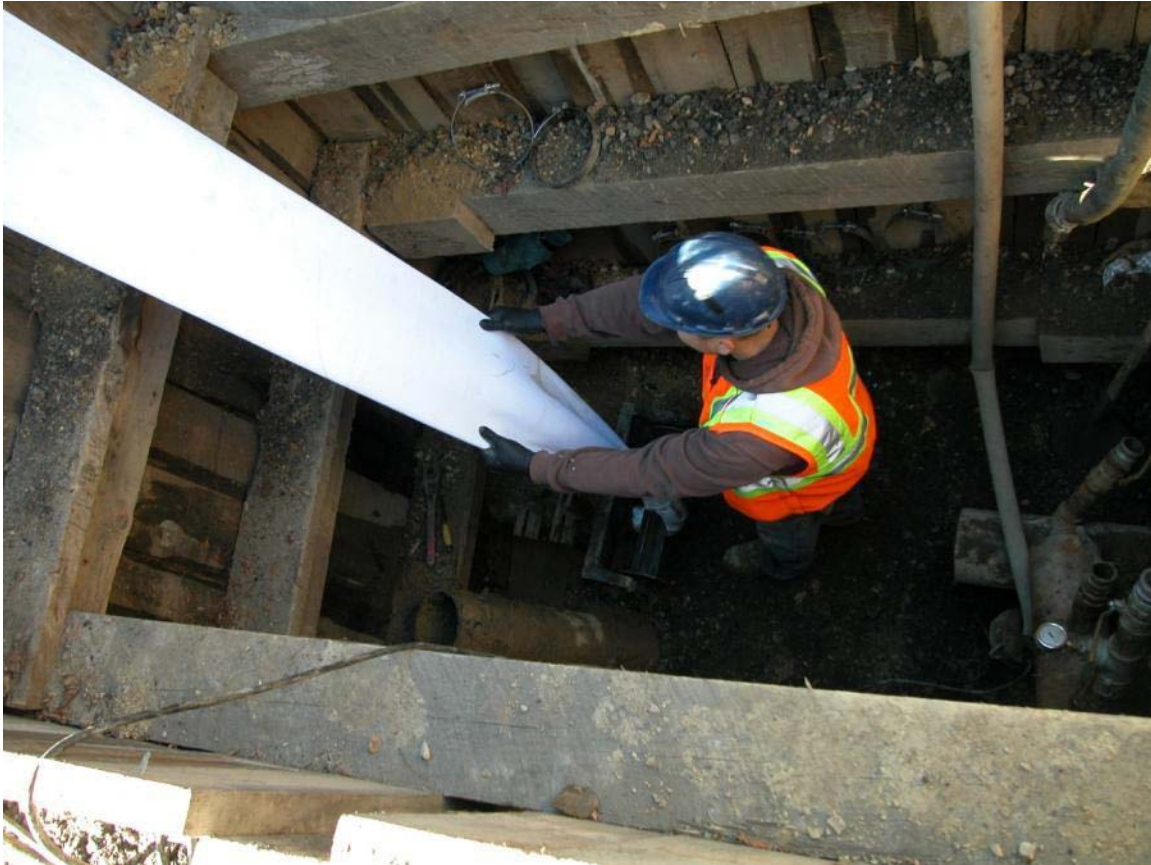
WATER MAIN LINING PROJECT ON DROSTER ROAD
