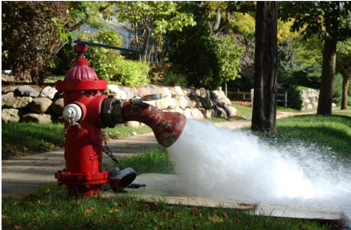
WATER MAIN FLUSHING IN PROGRESS
