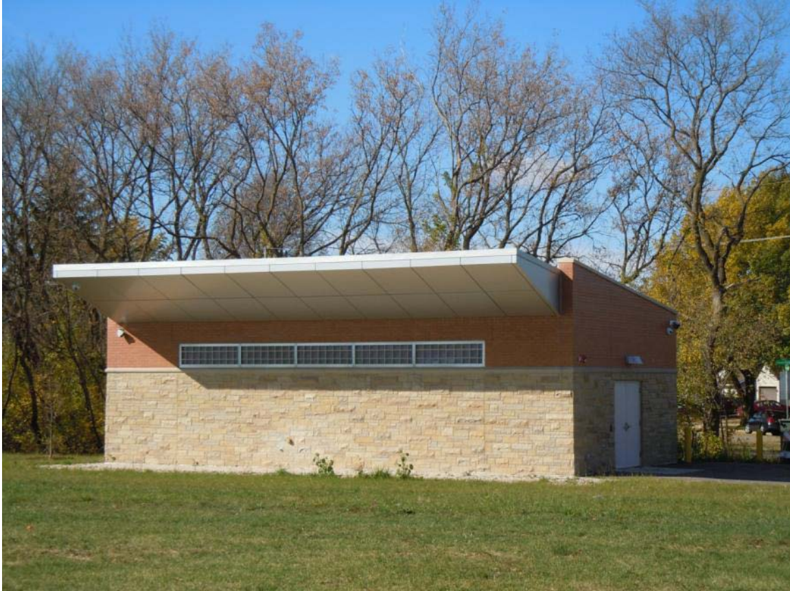
NEW BOOSTER STATION AT LEOPOLD PARK
