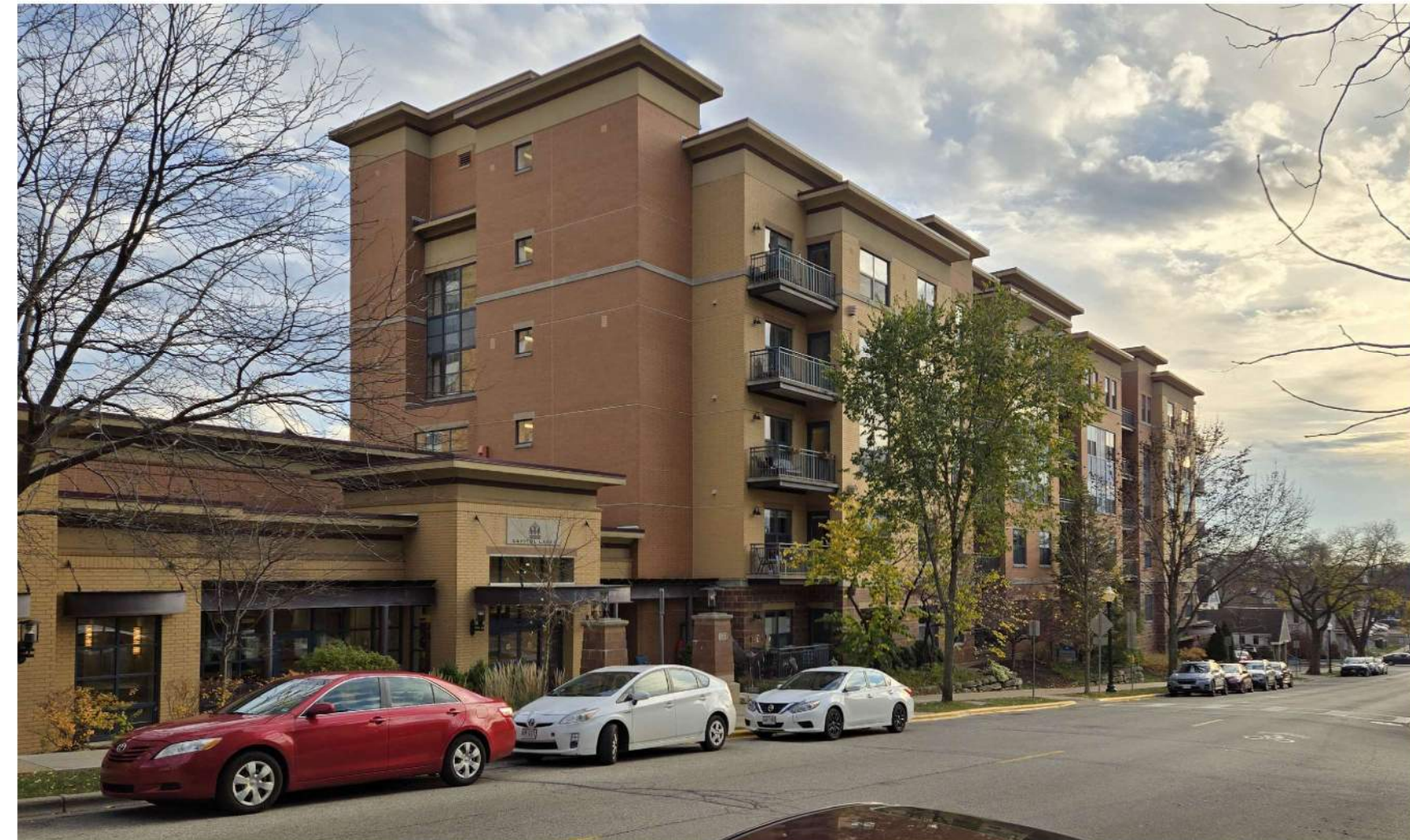
1: MAINGATE BUILDING - DOWNTOWN CORE
