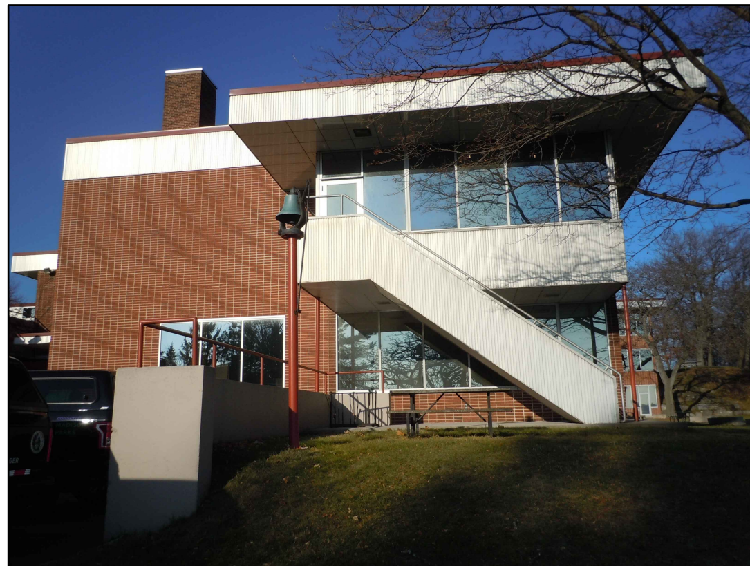
EAST FACE OF EXISTING BUILDING
