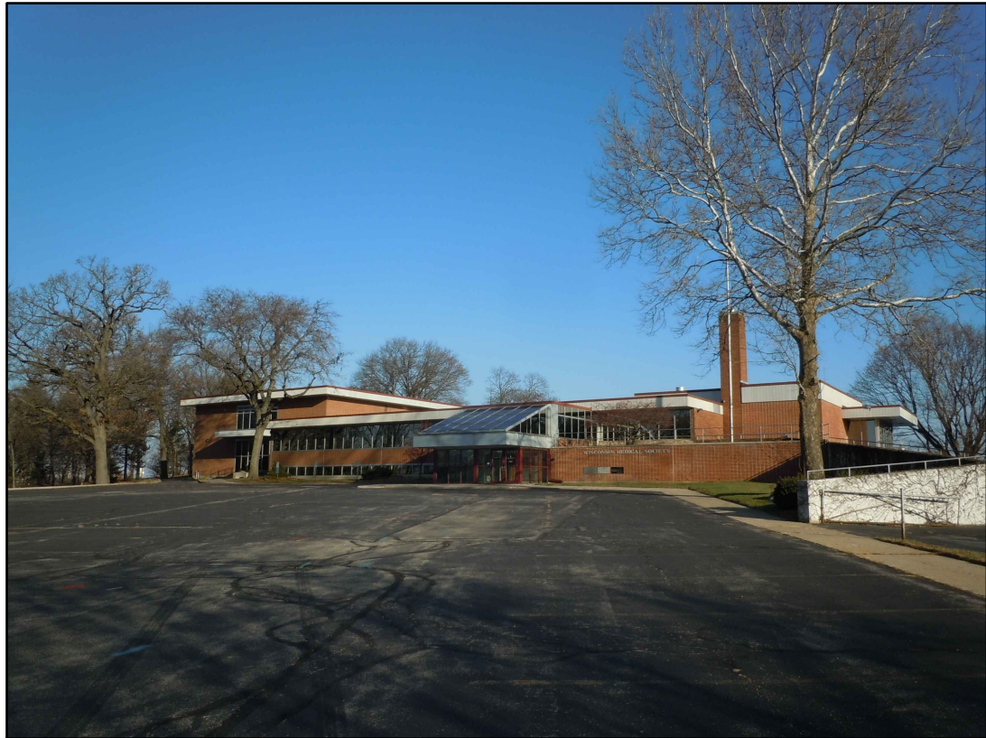
FACING NORTH TO EXISTING BUILDING
