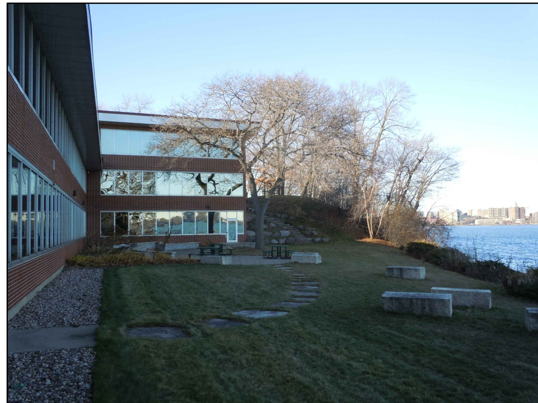
NORTH SIDE OF EXISTING BUILDING
