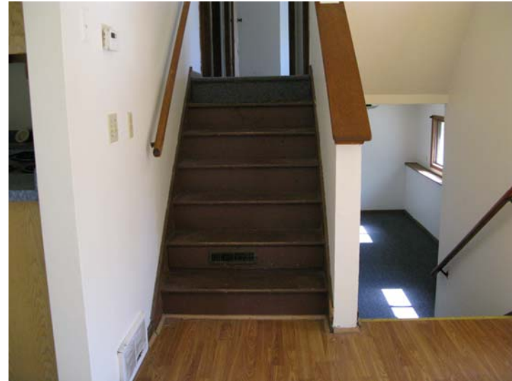
Unit 1411- Interior Showing Level Change
