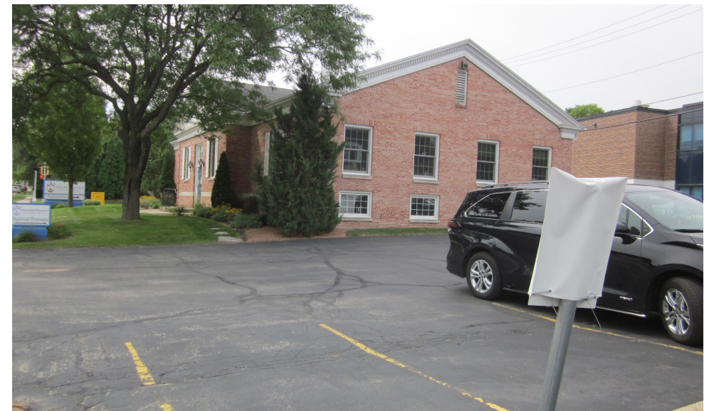
222 N Midvale Blvd Building Exteriors Site Demolition Images
