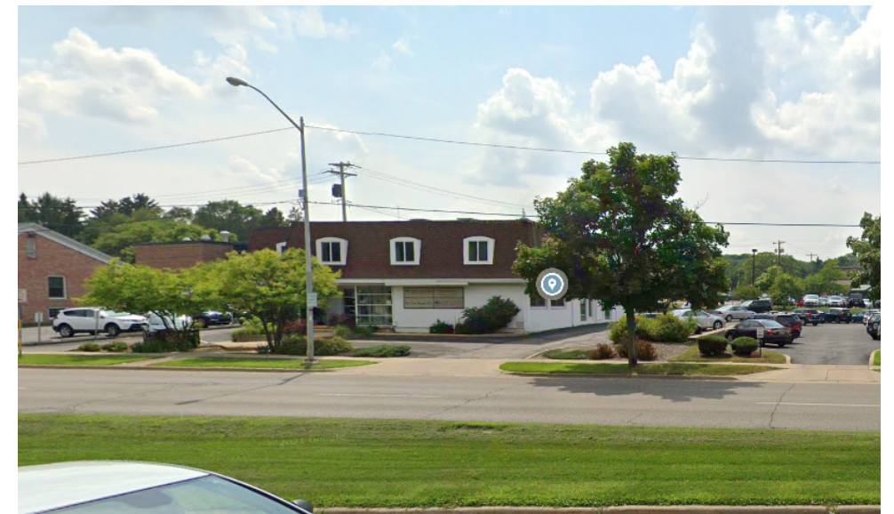
216 N Midvale Blvd Building Exteriors Site Demolition Images
