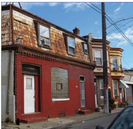
6.8 Buildings south of Frankford Ave.
