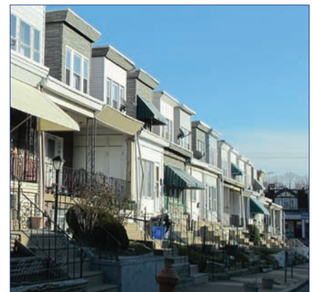
6.13 Grouping with low integrity
