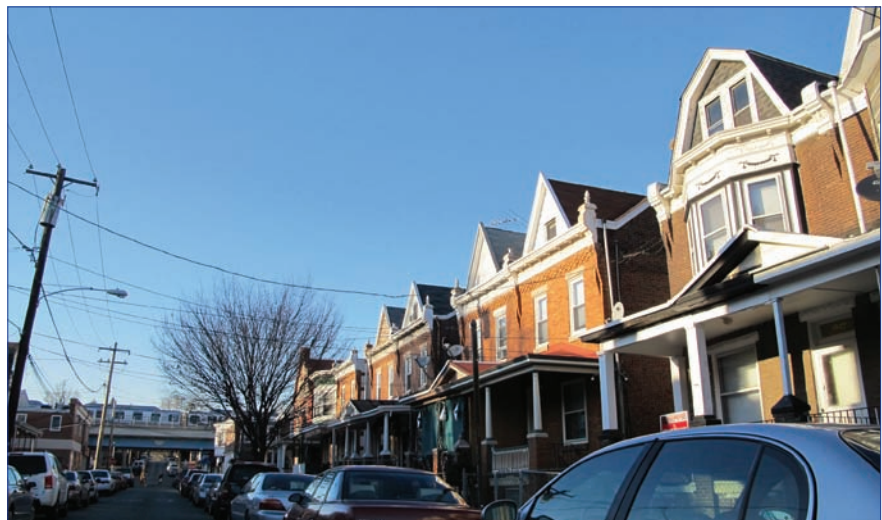
6.2 Block of high-integrity twins off Frankford Avenue
