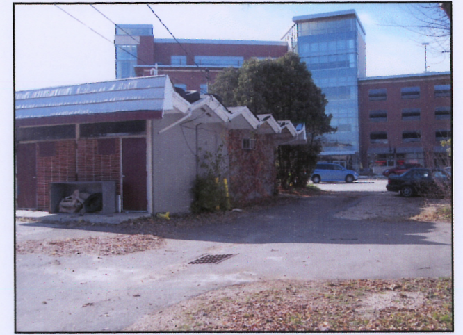
NORTHEAST CORNER OF LOT LOOKING SOUTHWEST
