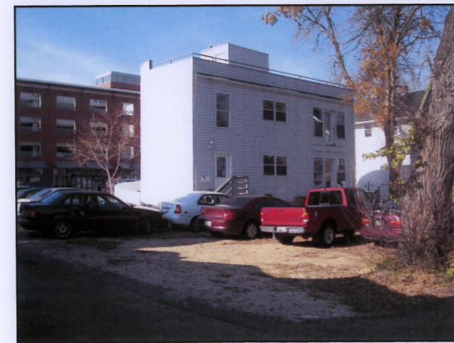
CENTER OF ALLEY LOOKING NORTHWEST
