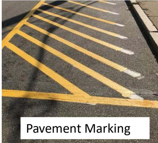
Buffer Zone will consist of pavement marking .
