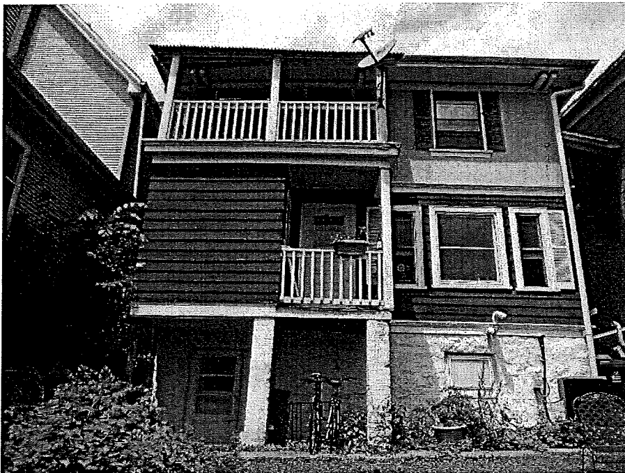
EXISTING BACK PORCHES
