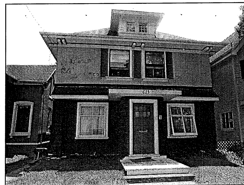
EXISTING NORTH WEST VIEW OF 625 E. GORHAM ST.
