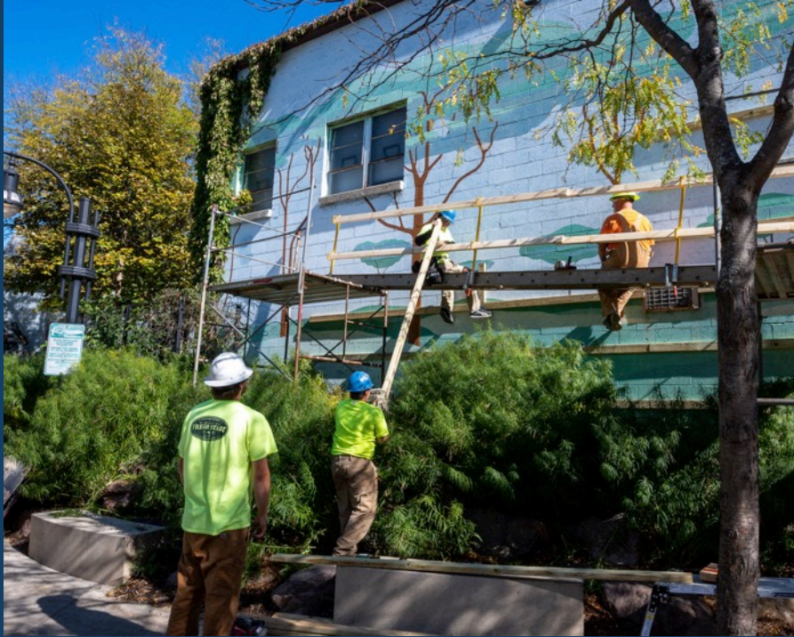
Operation Fresh Start student crew installing a mural with City of Madison
