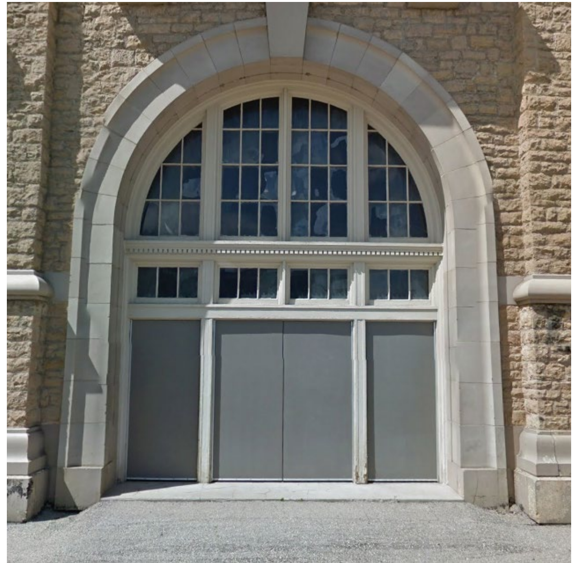
Typical door at original location South elevation
