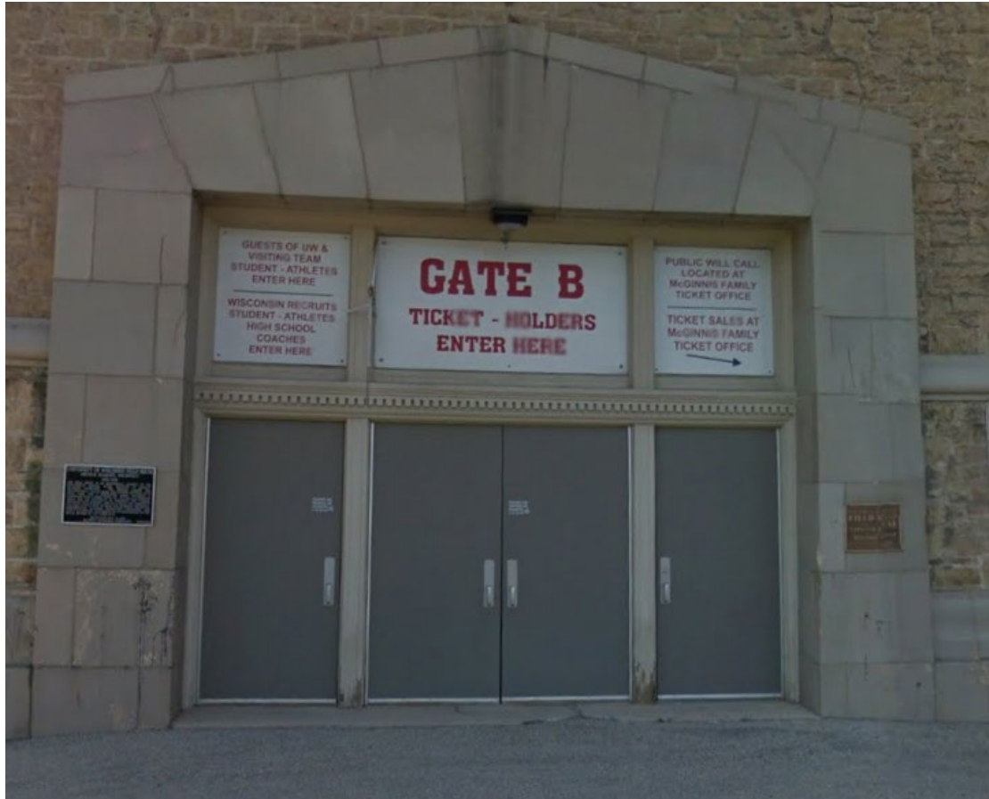
Typical door at original location East and West elevation
