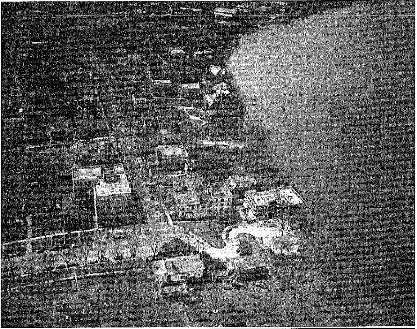
Edgewater Hotel under construction 1947.
