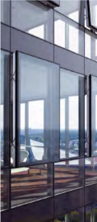
Glass Curtain Wall
