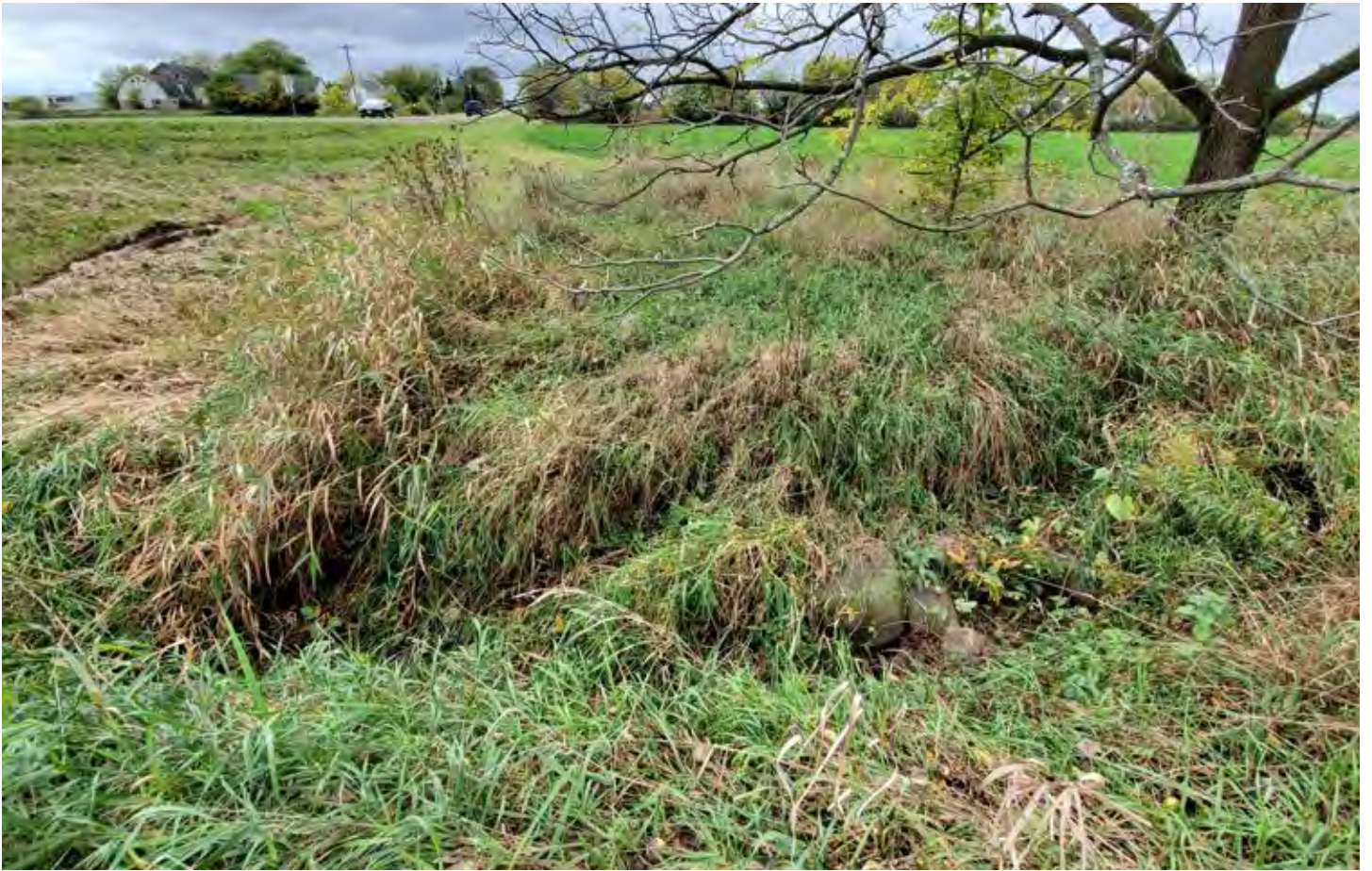
9- Standing near T5A facing west.
