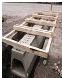
Figure 55. Photo. Construction and placement of amphibian tunnel in Waterton National Park, Alberta (Credit: Parks Canada).
