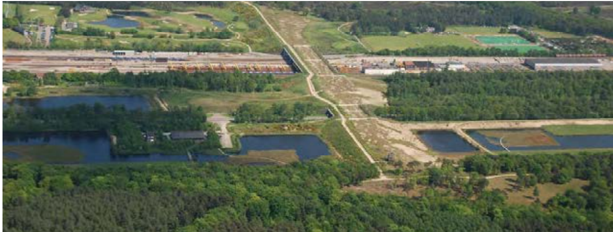
The Netherlands: Most wildlife overpasses or landbridges are less than 70-80 m (230-262 ft) long. The one shown above, near Hilversum, is 800 m (2625 ft) long and spans two roads and a railroad. (Credit: Goois Natuurreservaat, The Netherlands/Photo: W. Metz).
