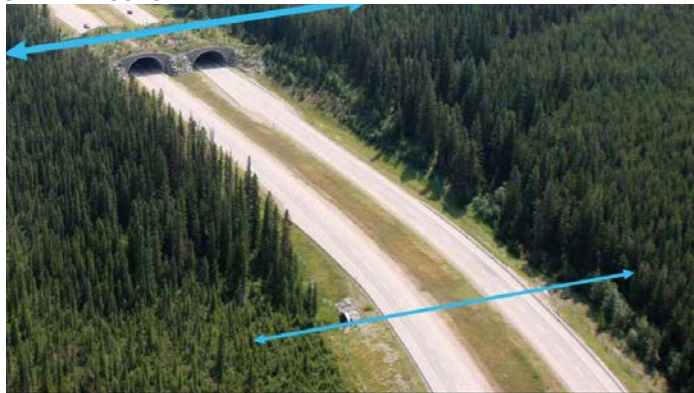
Landbridge and, at bottom, underpass (for critters that need underground passage)
