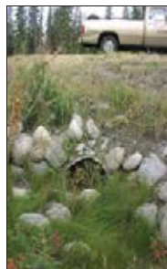
Figure 49. Photo. Small- to medium-sized mammal underpass (Credit: Tony Cleveger).
