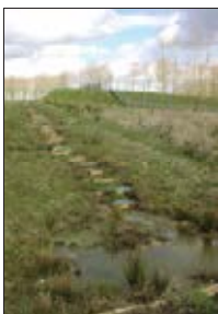
Photo. "Stepping stone" ponds on wildlife overpass used to assist amphibian movement (Credit: Tony Cleveger).
