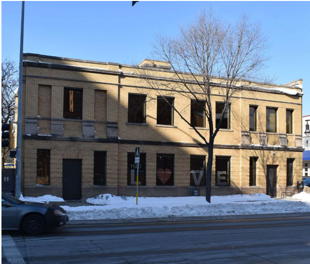
301 W JOHNSON STREET
