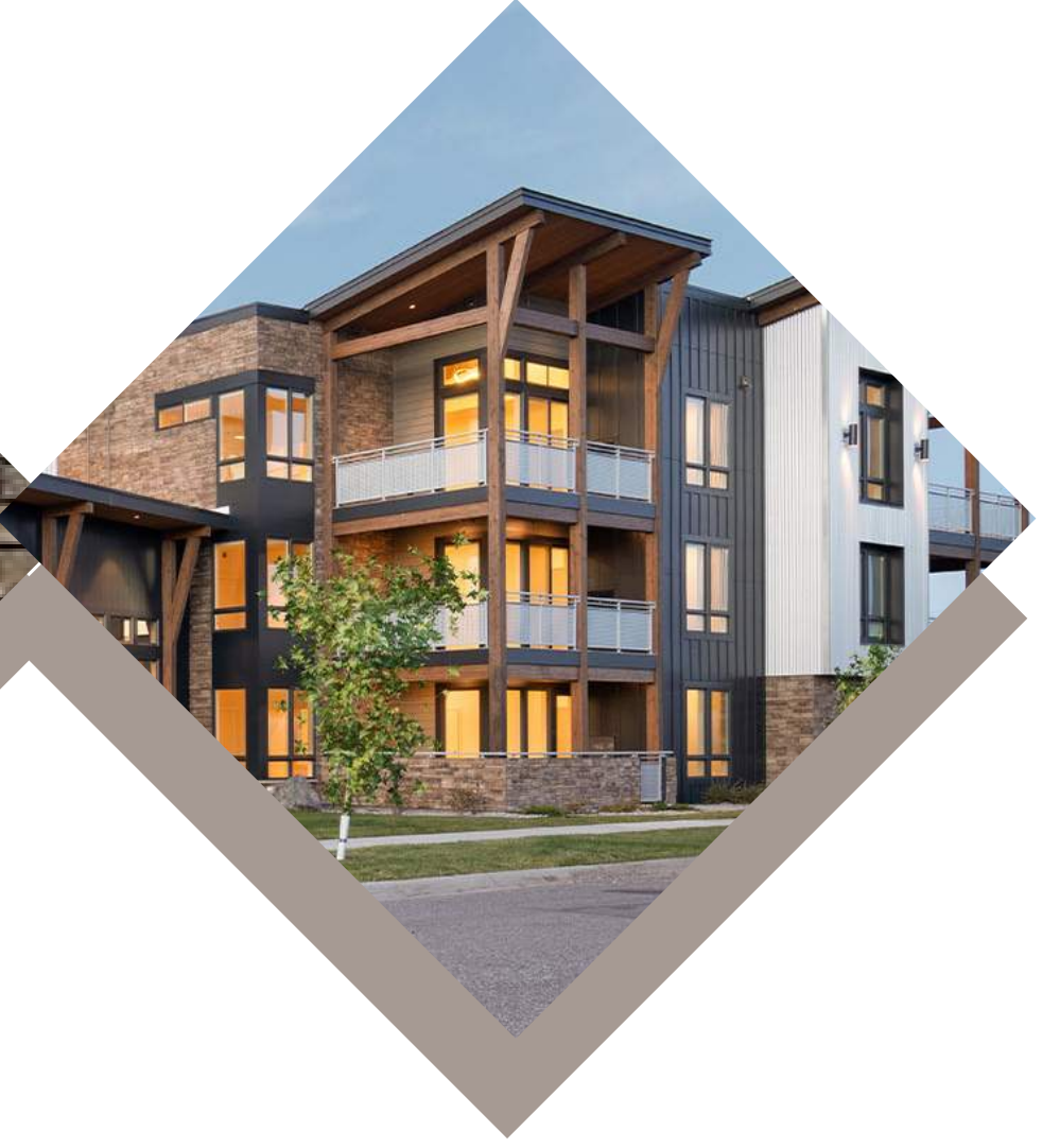
WOOD BEAMS & COLUMNS
