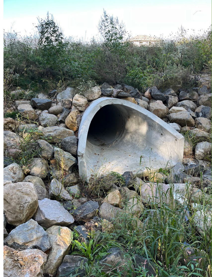
Outfall in dry weather
