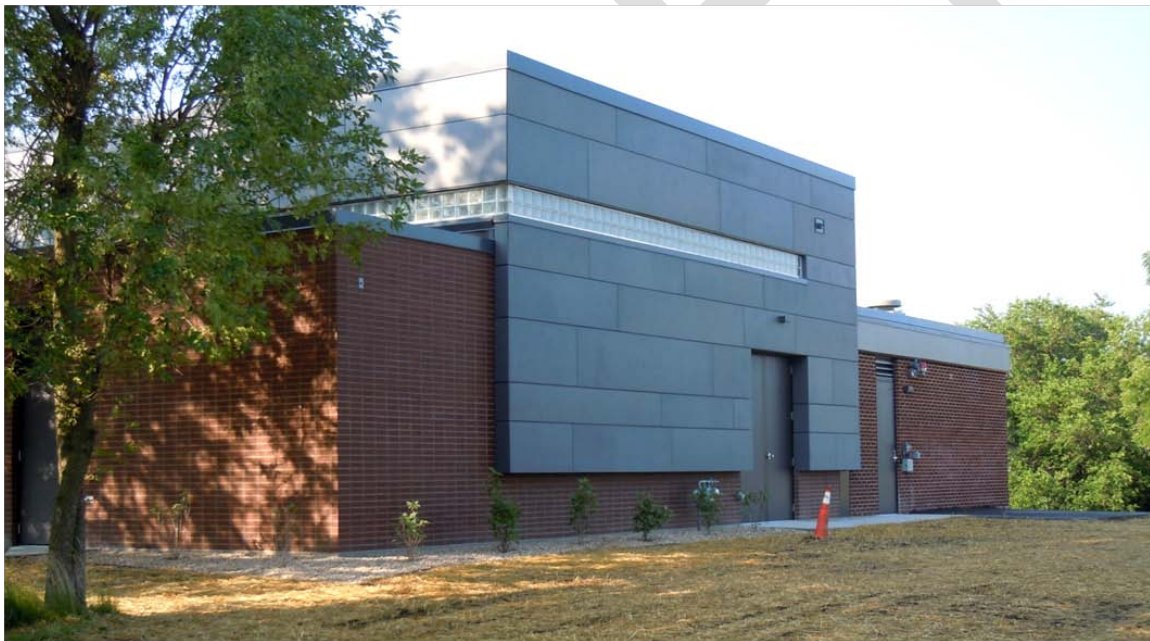
WELL 15 WITH NEW ADDITION TO HOUSE THE VOC AIR STRIPPER
