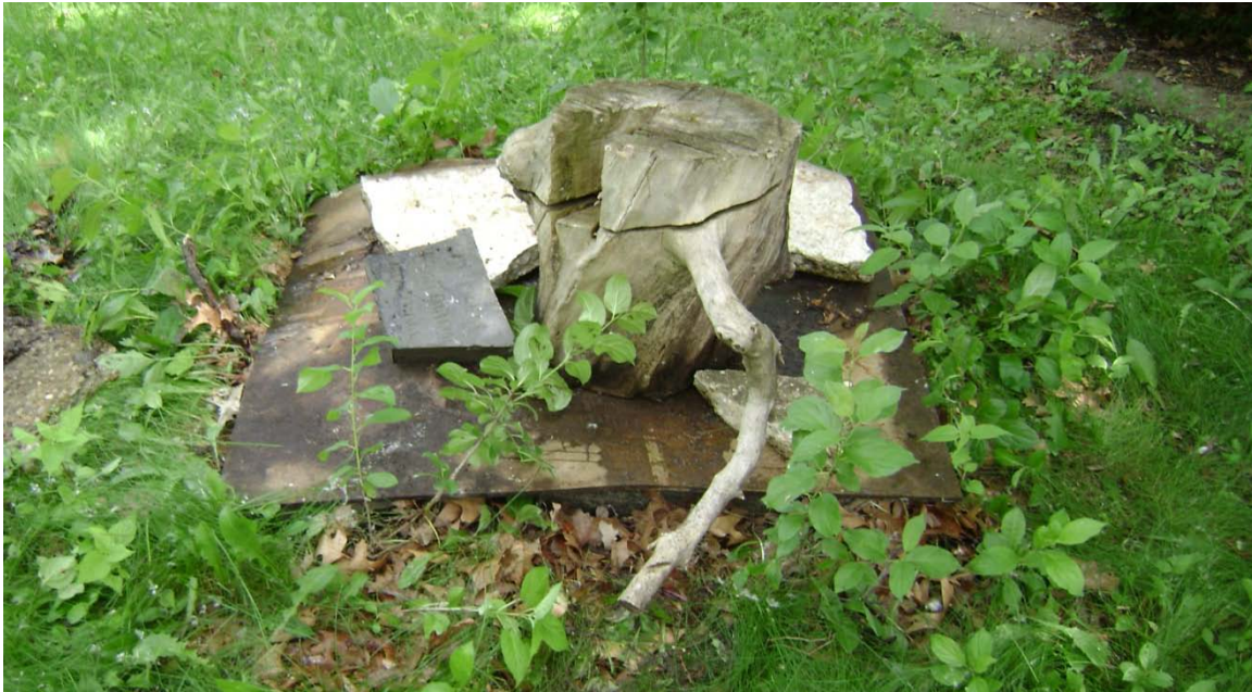
EXAMPLE OF AN UNABANDONED PRIVATE WELL FOUND IN MADISON
