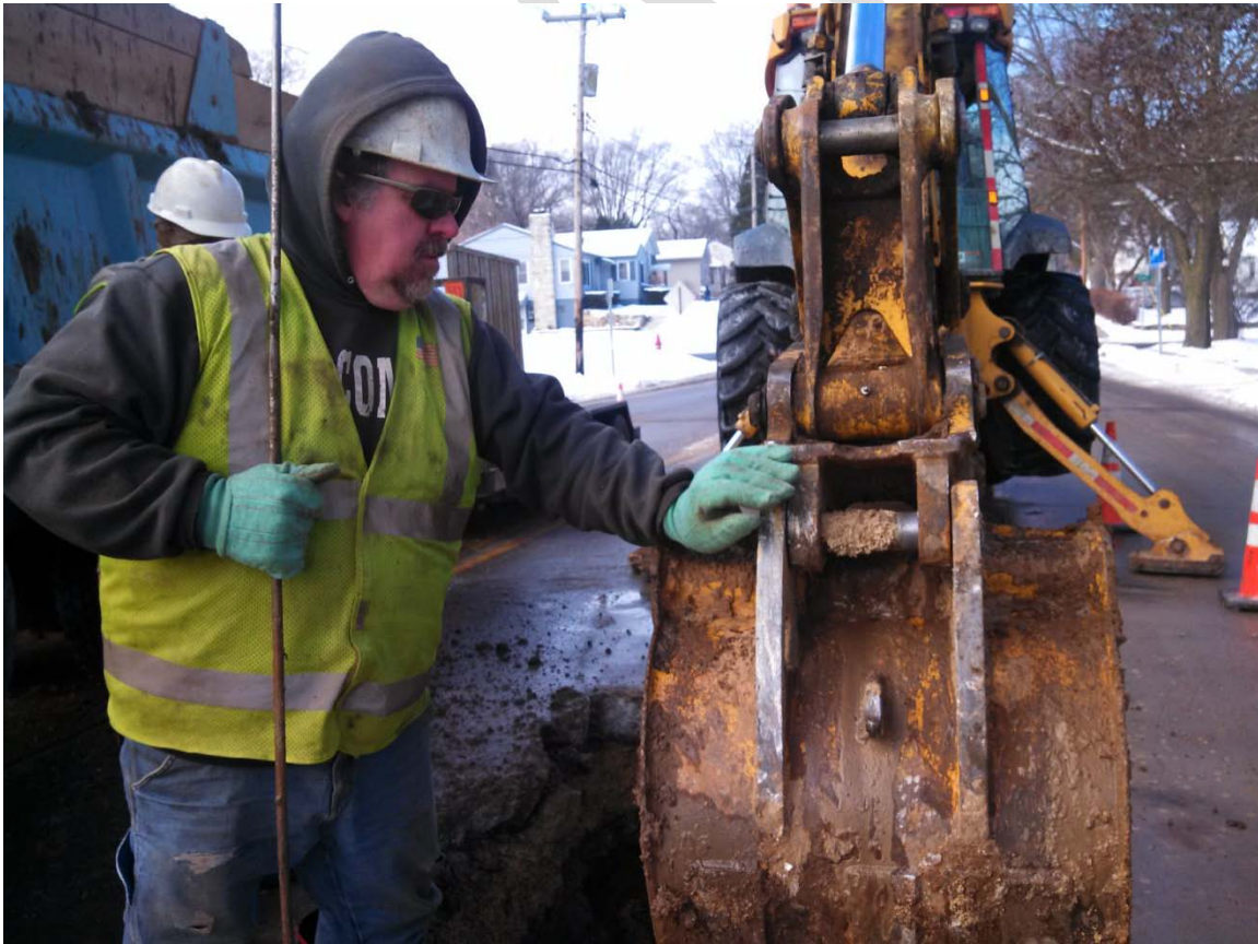
MWU CREW REPAIRING A WATER MAIN BREAK ON BUCKEYE ROAD
